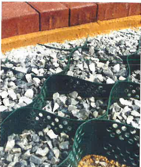
Fig. 2.7 Brick and gravel stabilizer system
