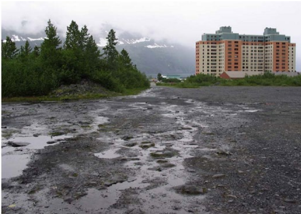
Figure 2. Seepage from Whittier Creek Dike flowing north towards the City of Whittier.
