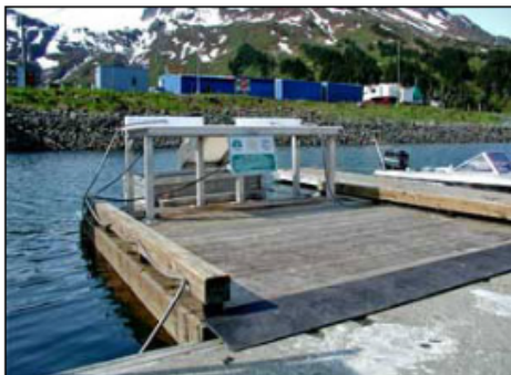
Cleaning table & dock #2 - View 1
