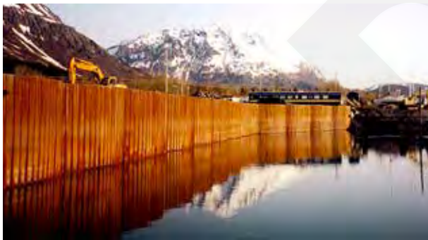
Sheet pile uplands expansion (Whittier and Seward)
