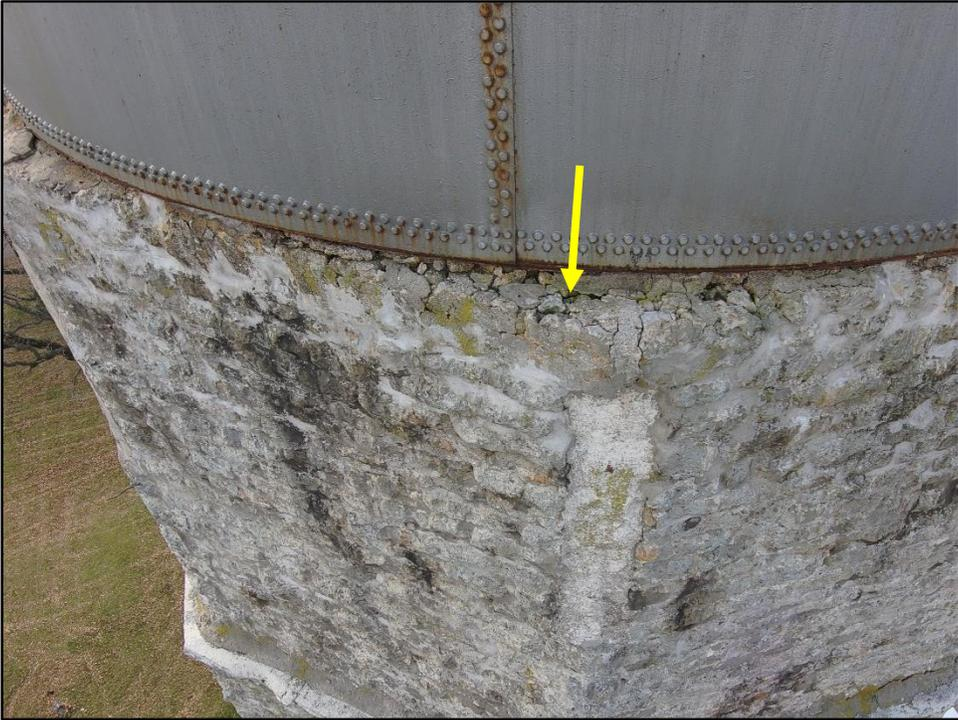
**Photo 17: Deteriorating masonry at top of wall**
