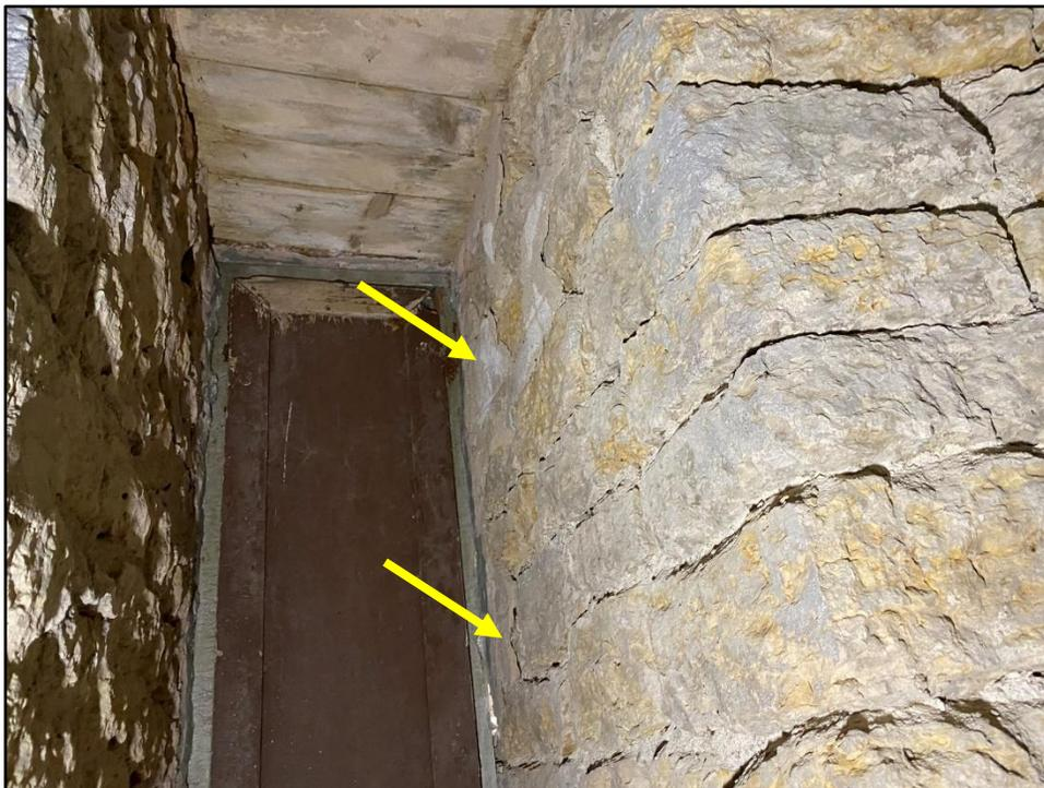
**Photo 19: Spalled stone on "door" walls**
