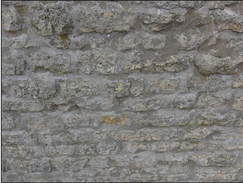
**Photo 26: Repointed joints at mid-height of tower**
