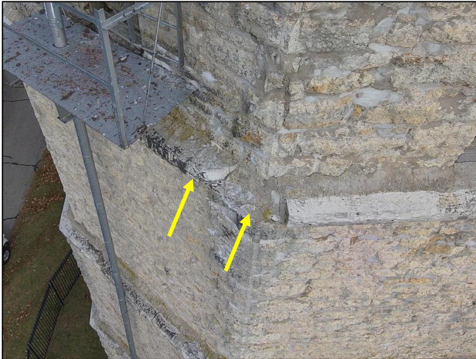
**Photo 15: Missing stone, cracked stone, deteriorating mortar wash**
