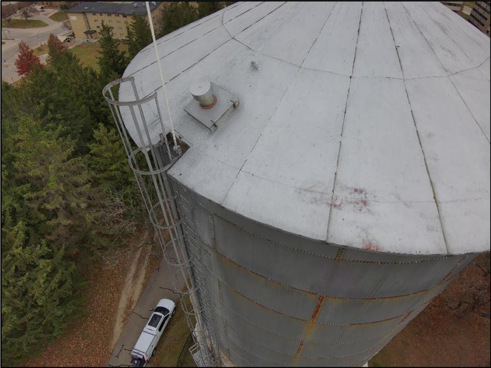
**Photo 9: Exterior ladder to tank**
