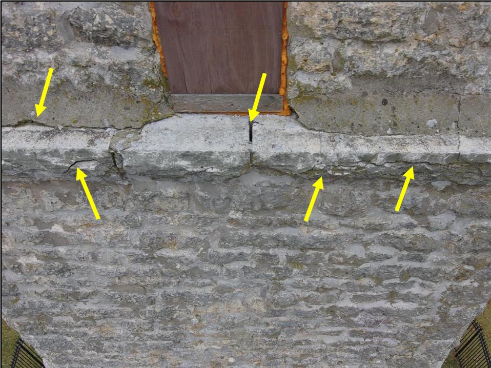
**Photo 14: Cracked stones, missing mortar, deteriorating mortar wash**
