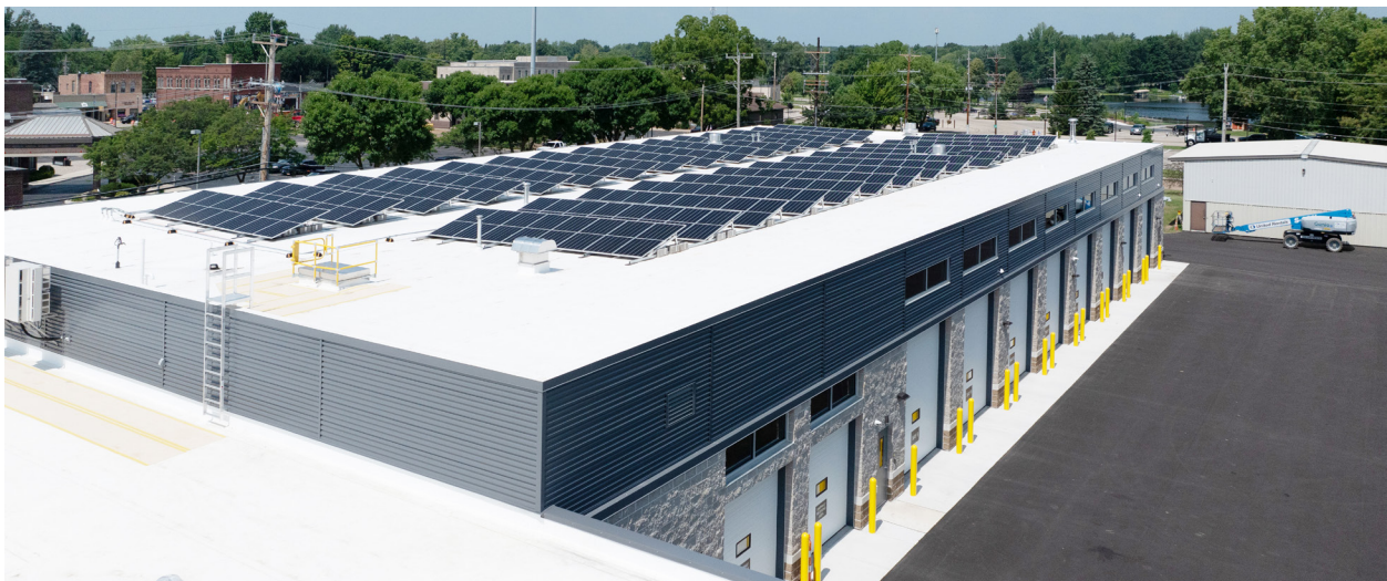
Shawano Municipal Utilities Garage – Shawano, WI
