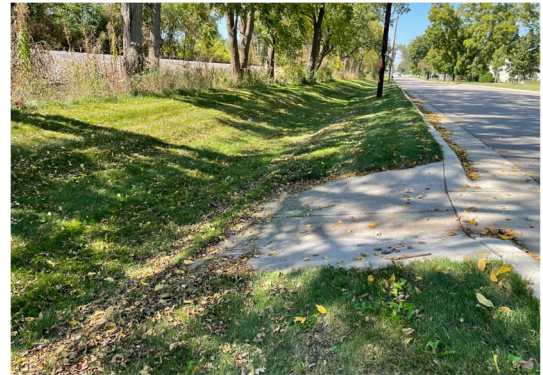
Curb cut and grass swale on East Main Street.
