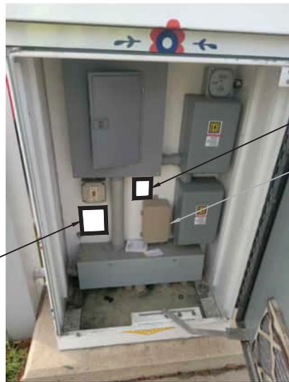
EXISTING LIGHTING CABINET NO SCALE
