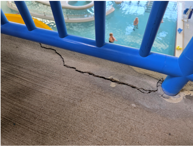
9. CRACKED/DETERIORATING CONCRETE
