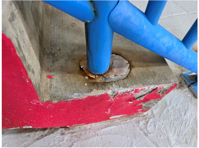
8. CRACKED/DETERIORATING CONCRETE
