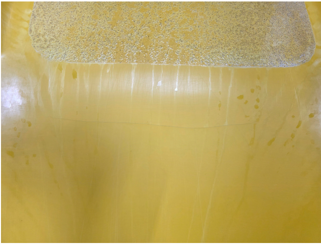
13. SCRATCH IN THE FLUME ENTRY TUB
