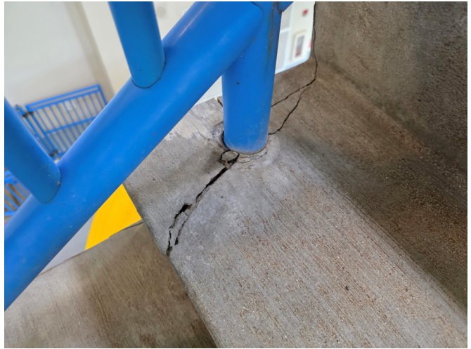
10. CRACKED/DETERIORATING CONCRETE
