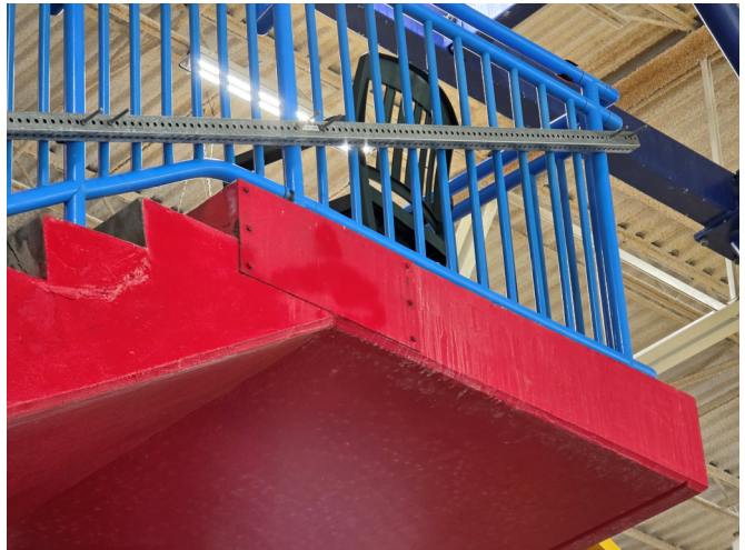
12. STRUT INSTALLED TO SUPPORT RAILINGS
