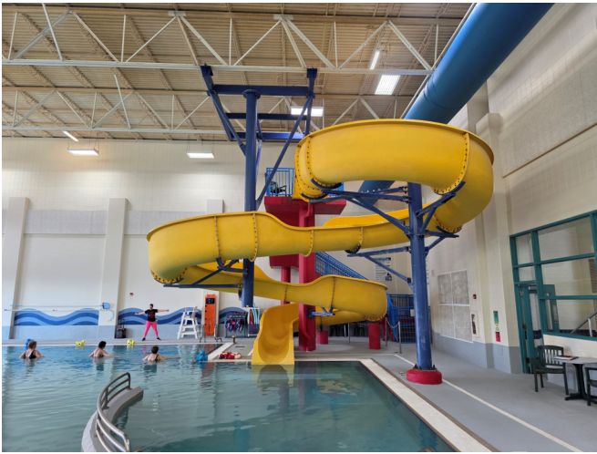
1. OVERALL VIEW OF THE SLIDE
