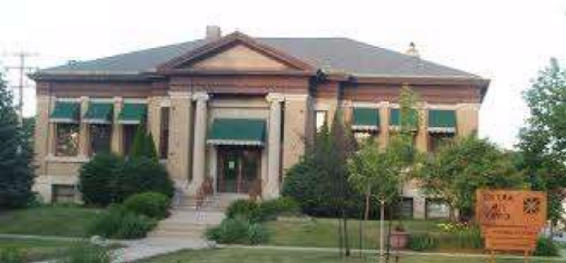
White Memorial Building, 1904 (present home of Whitewater Arts Alliance & City of Whitewater's Cable TV Station)
