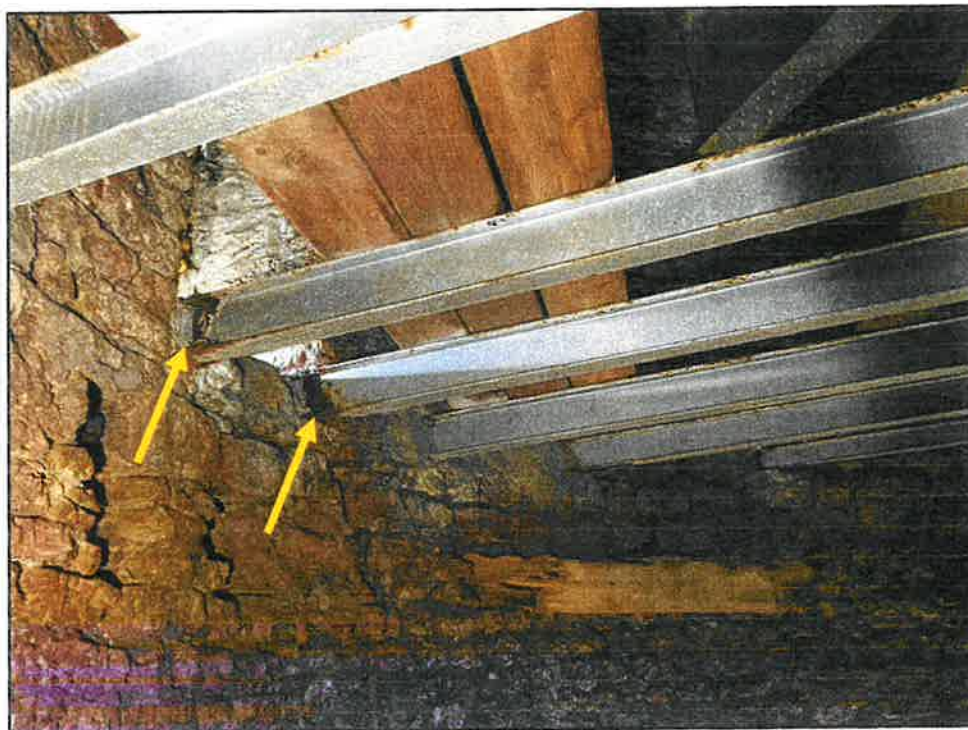
Photo 34: Signs of floor beam corrosion at walls
