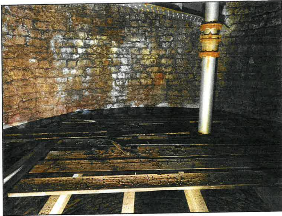
Photo 4: Floor below tank at top of masonry tower
