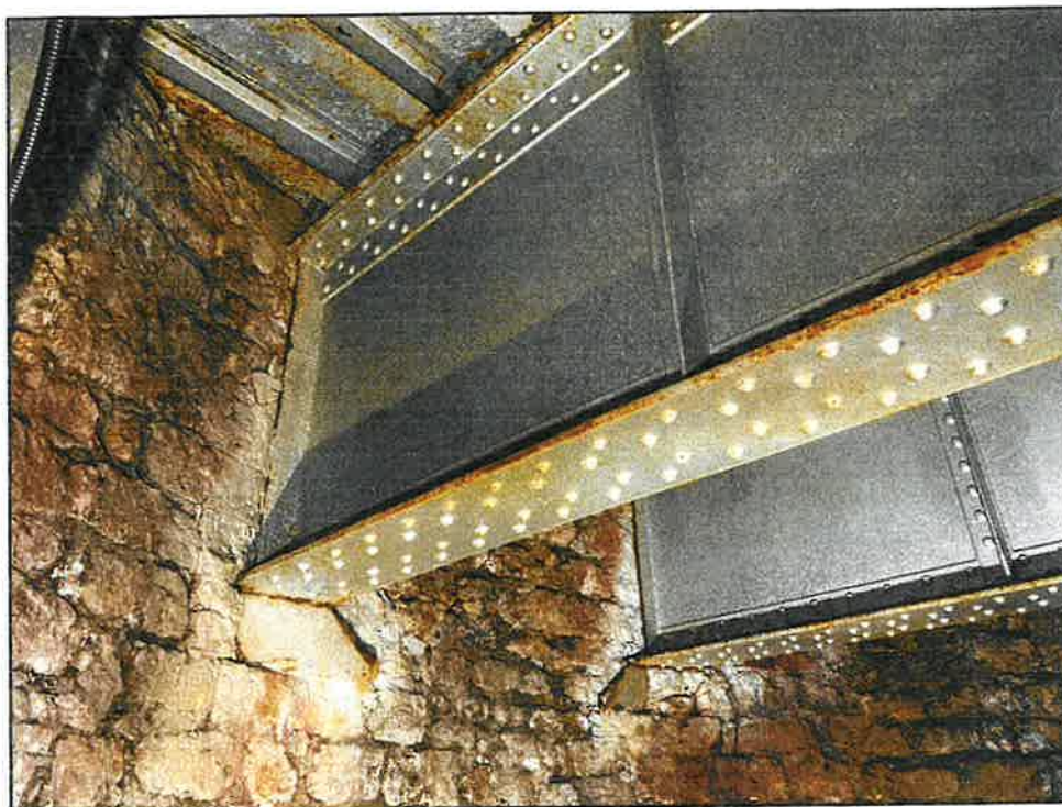
Photo 31: General light corrosion on support structure
