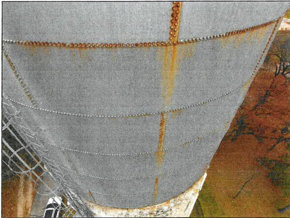
Photo 36: Rust staining on exterior of tank
