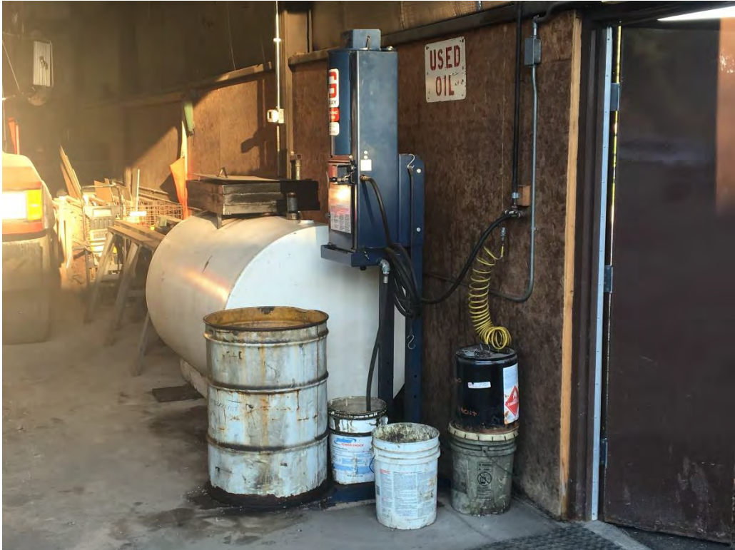
Looking Northwest at Used Oil Tank and Used Oil Filter Container
