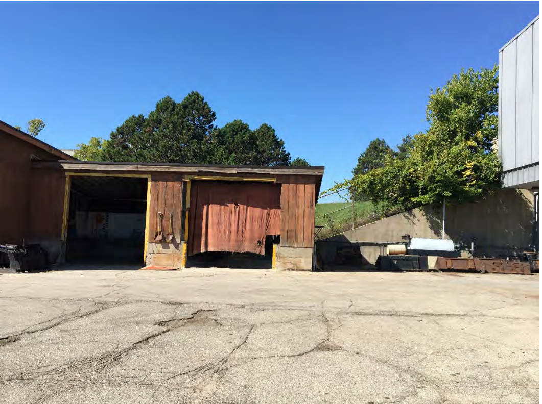
Looking west at salt storage shed.
