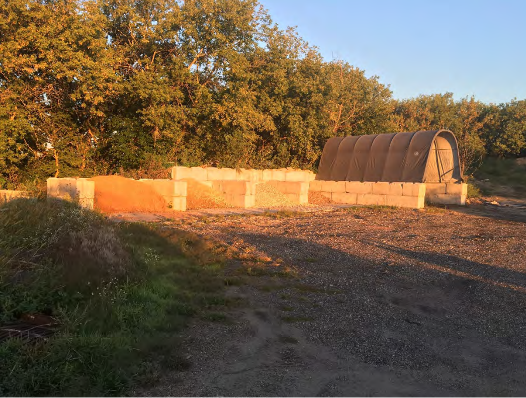
Looking Northwest at gravel storage areas.
