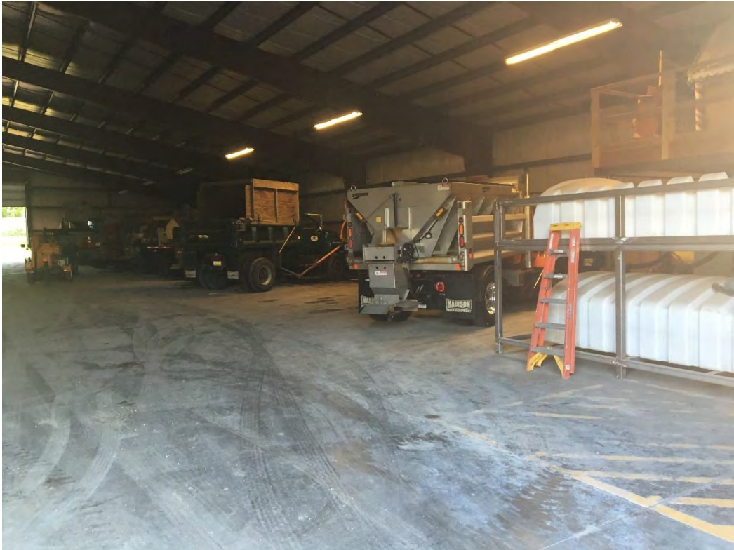
Looking Northeast in Cold Storage Building
