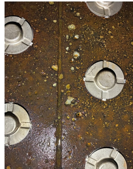
Figure 4 Underdrain Plate Pitting
