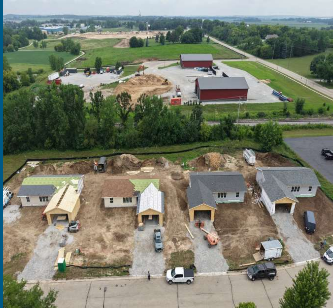
Stonehaven single-family homes rising on Bluff Road, with the Tanis industrial condominium development and the Summerset Marine site beyond — Goals 1 and 3 in a single frame.
