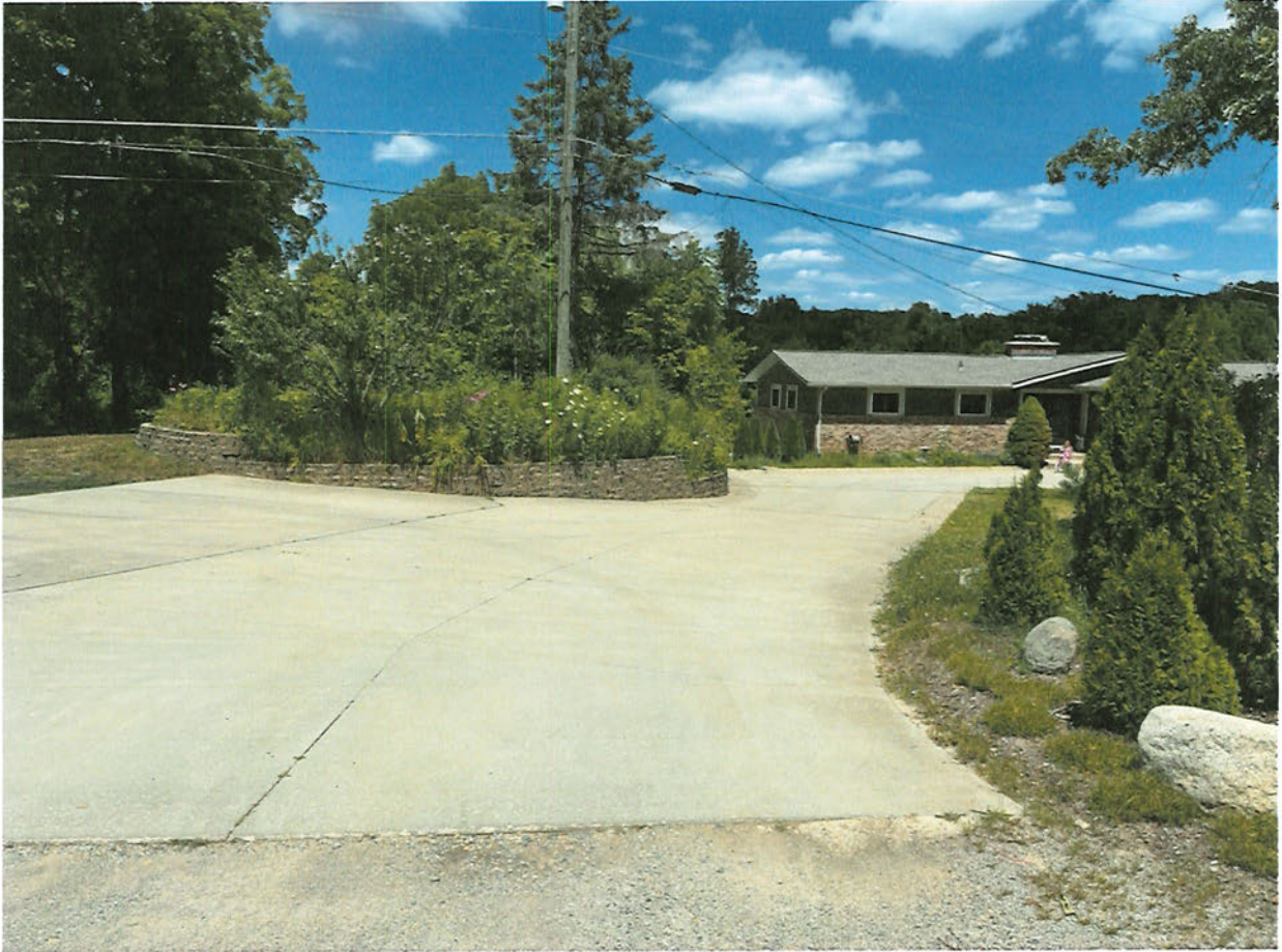
Figure E-2 – Concrete Driveway Entrance
