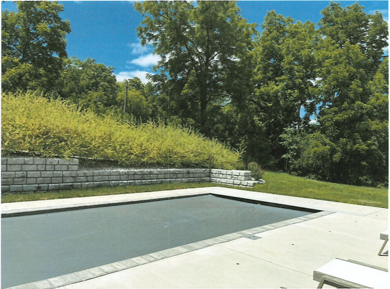
Figure C-1 – Overall View of the Pool Area
