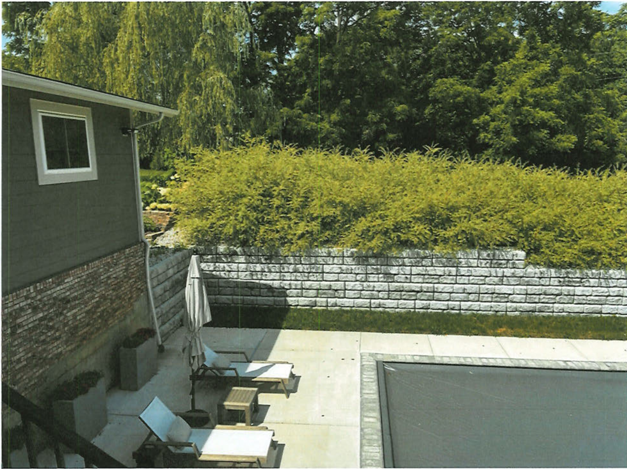
Figure 9 – Retaining wall and improved pool surroundings.
