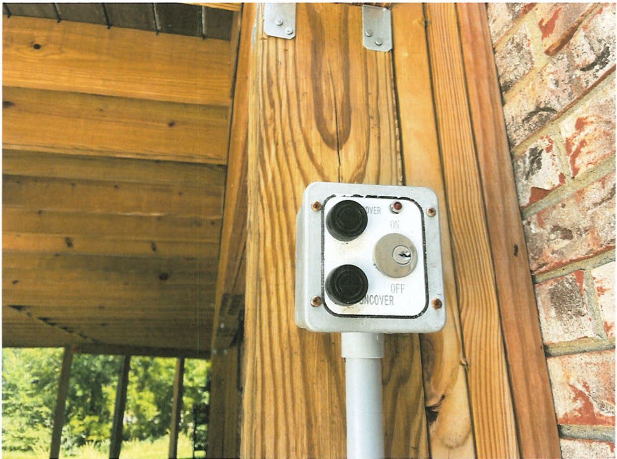
Figure D-2 – Keyed Control Switch (Key Removed)
