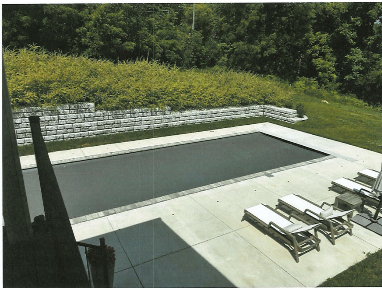
Figure 8 – Automatic safety cover secured over the pool.
