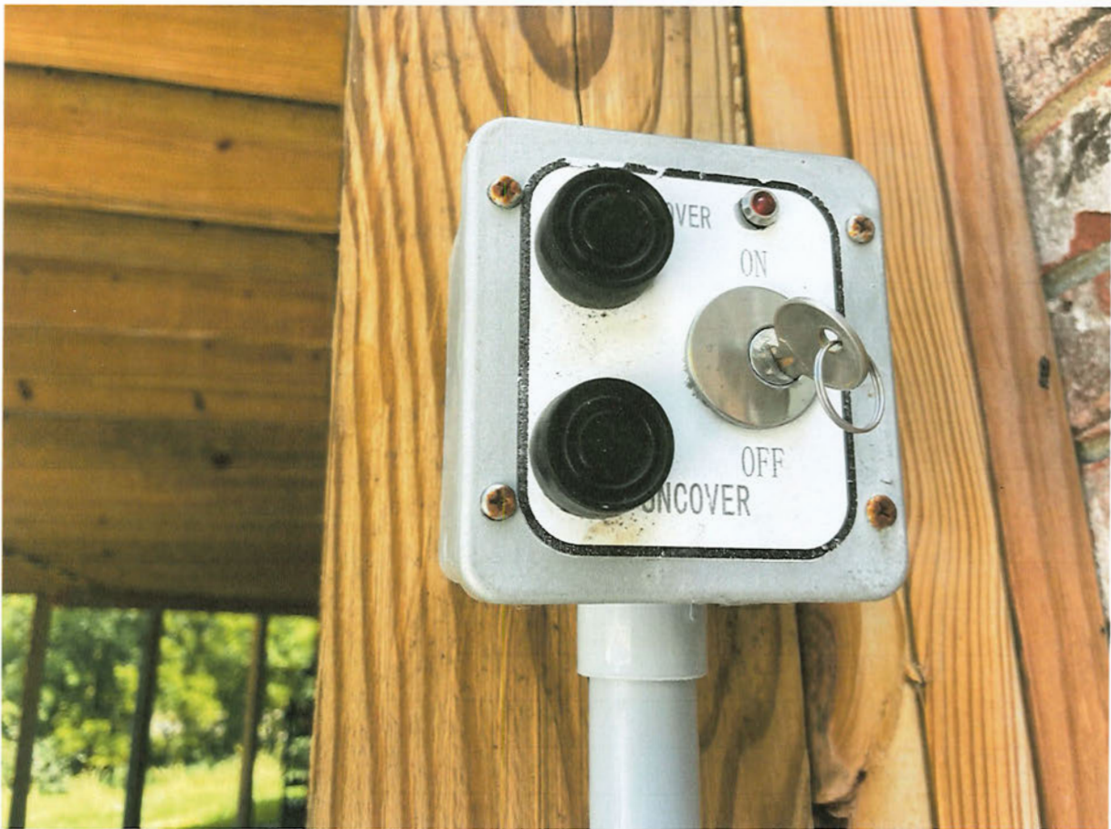
Figure D-1 – Keyed Control Switch (Key Inserted)
