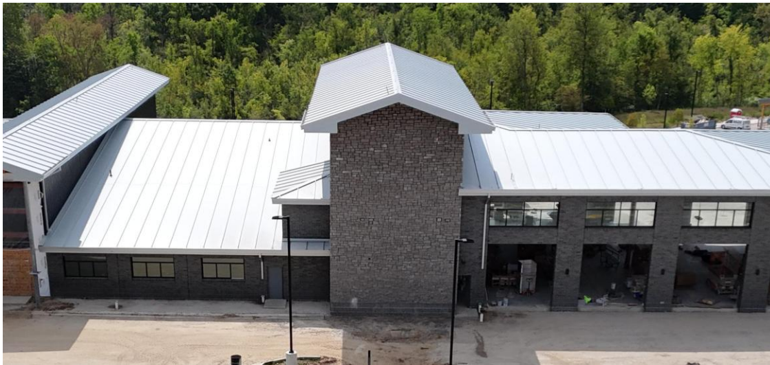
New Public Safety Building — brick installation complete on the hose tower wall (8/21/26)
