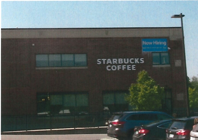
EXISTING SCOPE OF WORK: FRONT ELEVATION - REMOVE AND INSTALL NEW STARBUCKS DISK. Existing: 42" x 14' = 49 sqft
