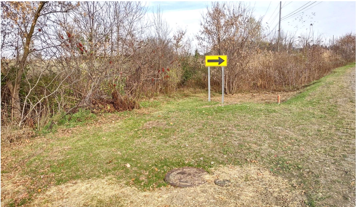
PHOTO 2 – Southeast Side, Near Culvert Crossing – Looking North
