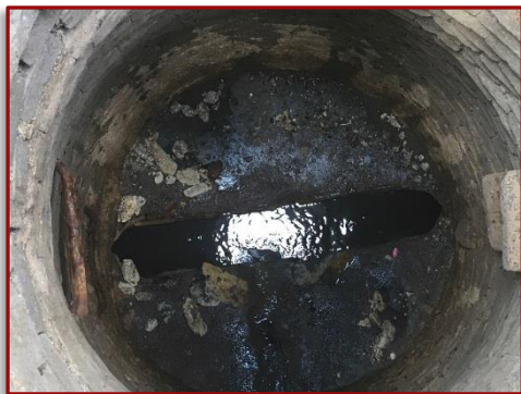
Wastewater Manhole Structure
