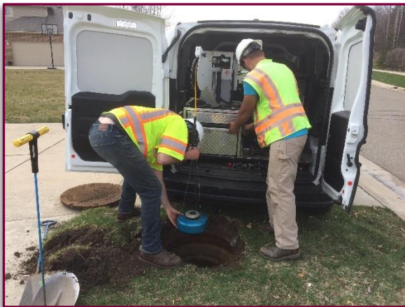
Figure 20 Manhole Scanning
