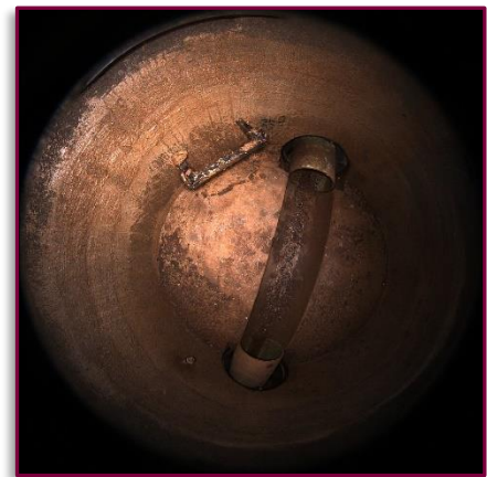
Wastewater Manhole Structure
