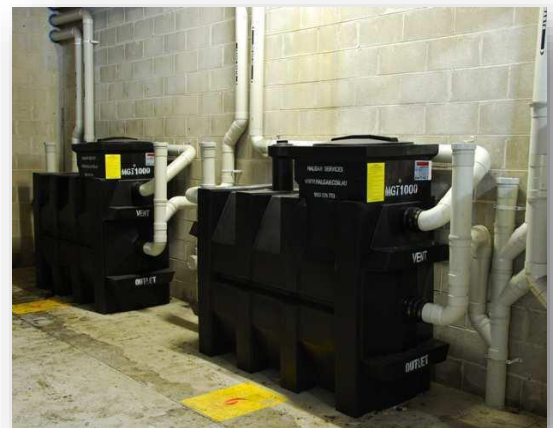
Grease Interceptor (In Basement) Example
