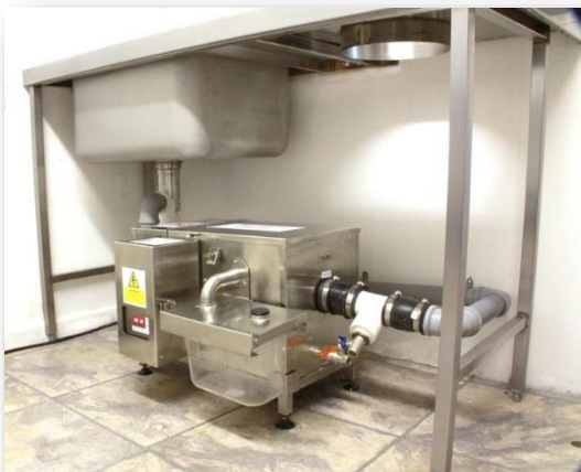
Grease Trap (Under the Sink) Example
