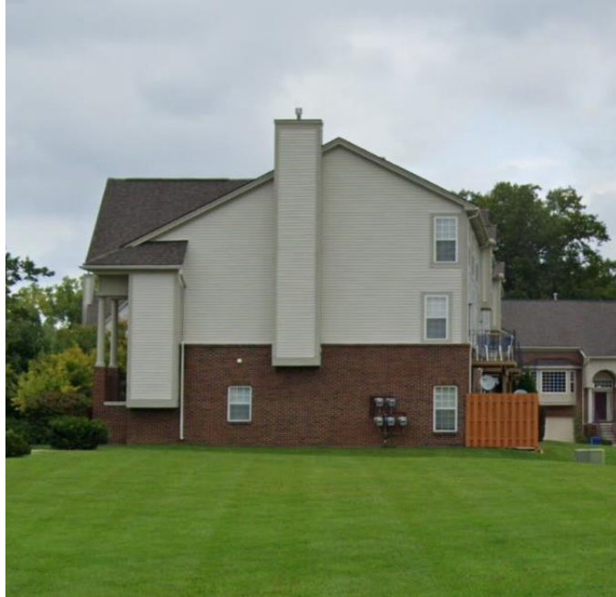
Existing Condominium Building
