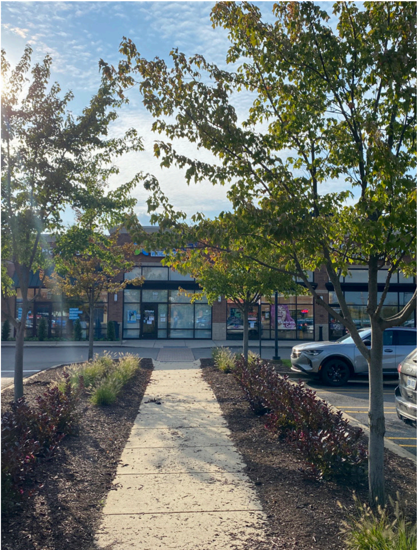
Sidewalk in commercial development
