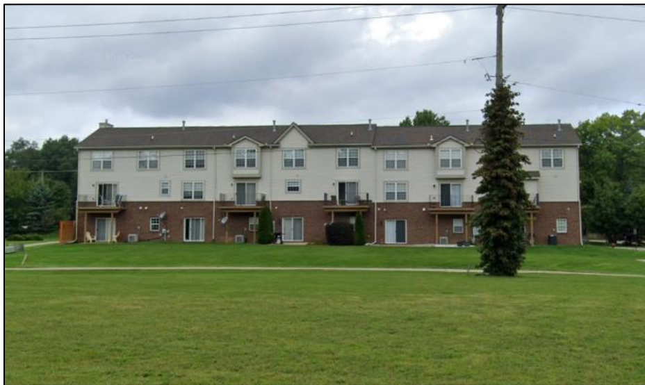
Existing Condominium Building
