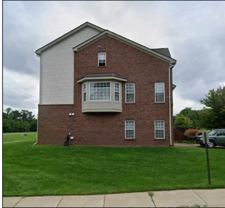
Existing Condominium Building
