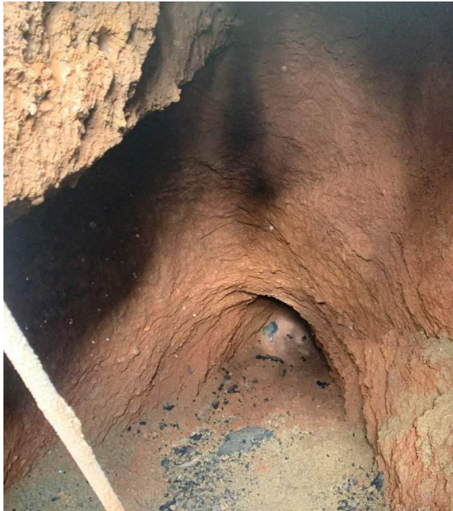
Photo 5: Brick Exposed at End of Tunnel
