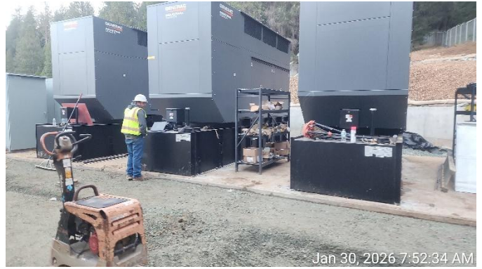
Installing Pipe Supports inside Pump Station
