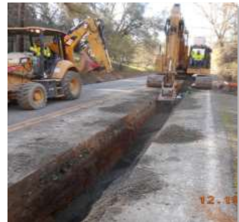
EID, Town Center Force Main Replacement, 2018
