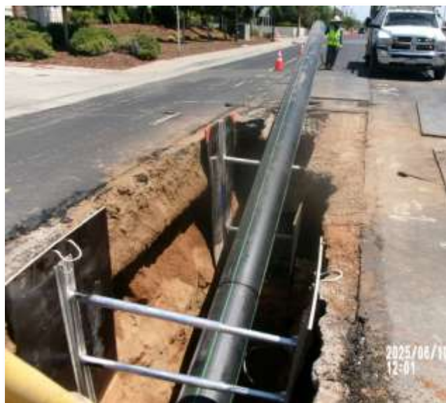
CCCSO, Lafayette Sewer Renovations, current
