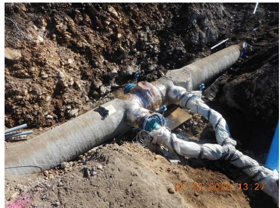
Cathodic Protection Wrap of Valves at Canchulagua
