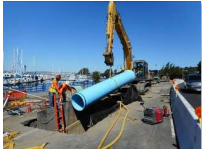
VFWD, Mare Island Way Sewer Rehabilitation Project, 2019
