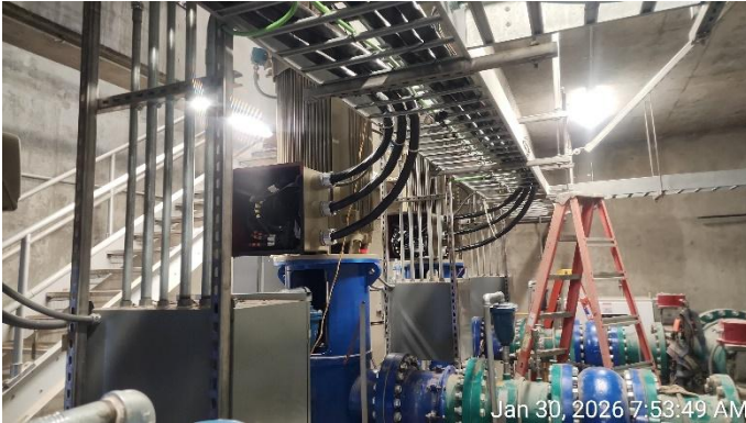
Landing Power Cables to Pump Motors
