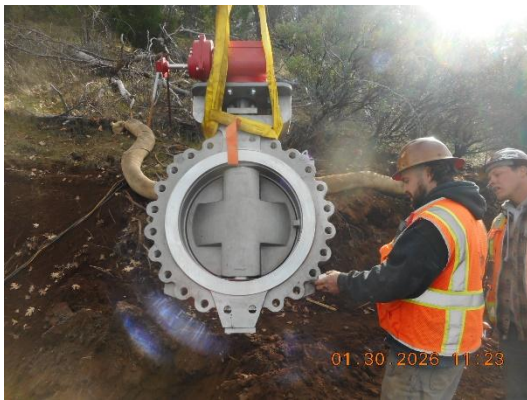
Installing 24" Butterfly Valve at Station 335+98
