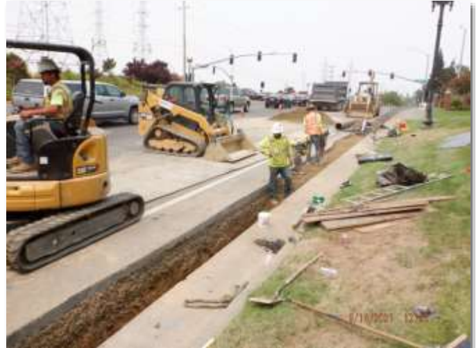
City of Folsom, Oak Avenue Wastewater Pipeline Project, 2023
