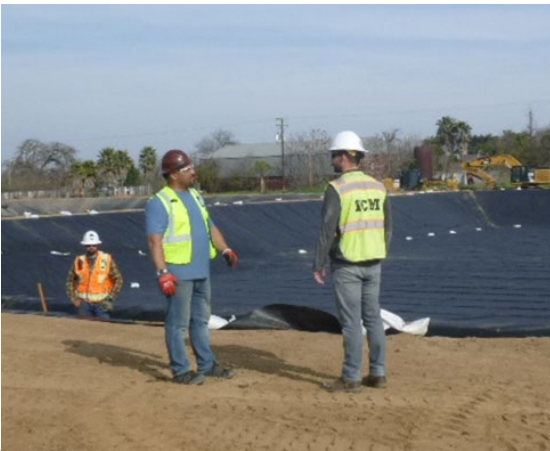
ICM employee talking with Contractor at the SJWD Hinkle Reservoir Project, 2023
