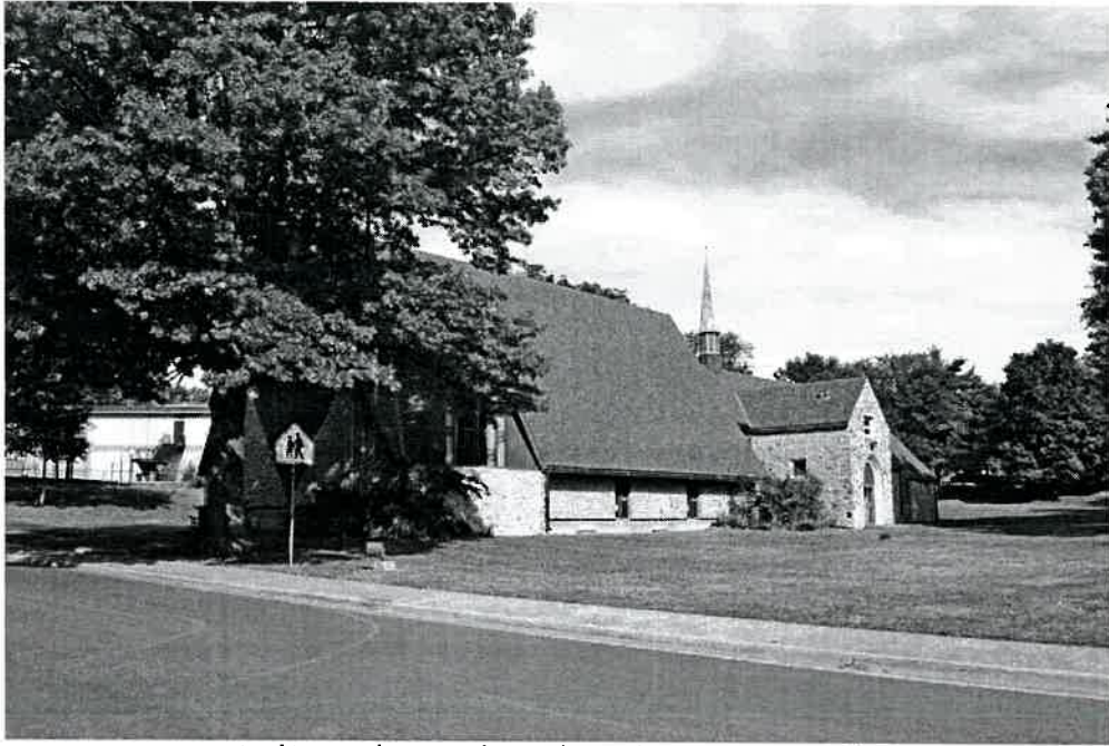
Looking northwest at the southeast elevation of the building
