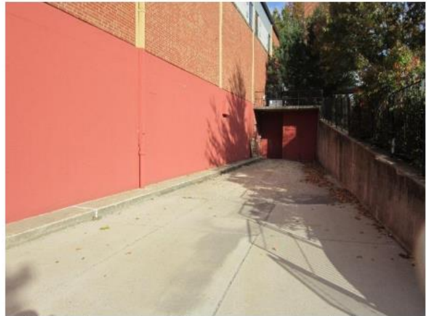
Additional exterior lighting recommended for security.
