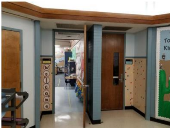
Classroom door recess
