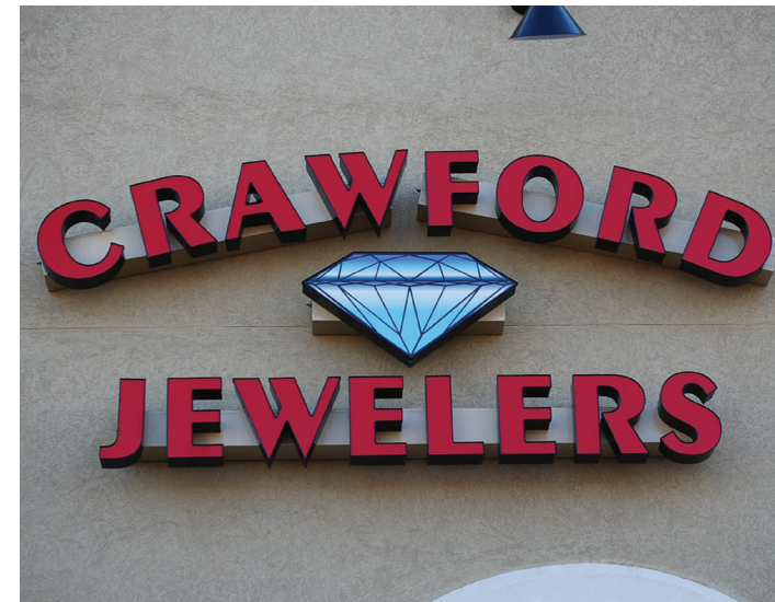
Exposed raceways, heavy trim cap
