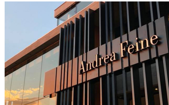
Fabricated letters integrated into architecture
