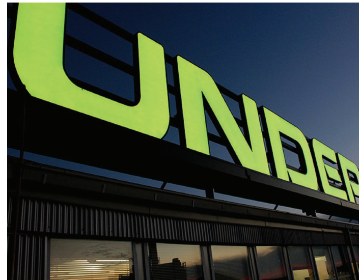
Internally illuminated signs with plastic faces
