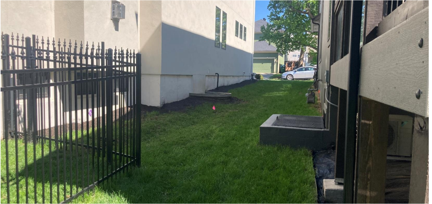
Western border looking North
