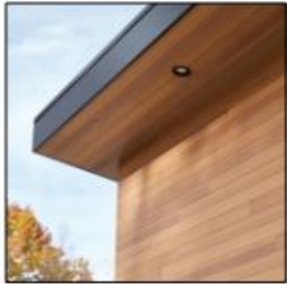
205: WOOD-LOOK SOFFIT AND SIDING
