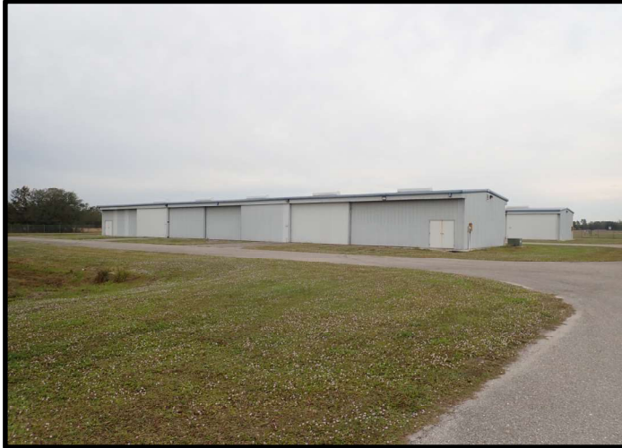
Photograph 1 - Overall view of hangar.
