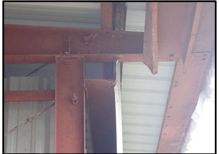
Photograph 4 - Missing purlin.
