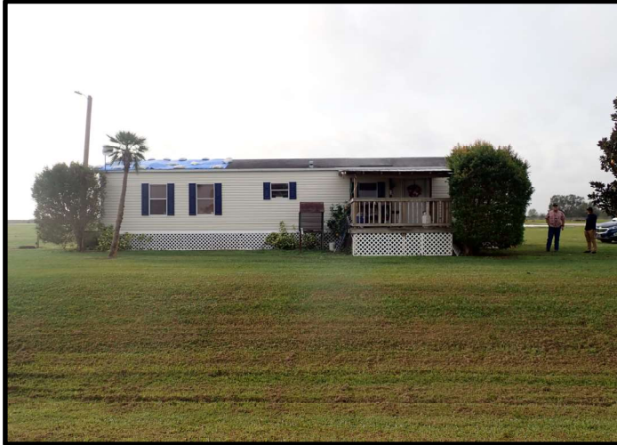
Photograph 1 - Overall view of building exterior.
