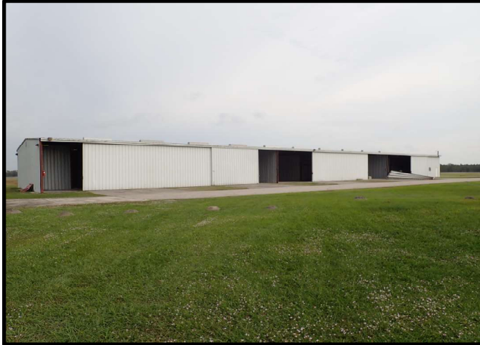
Photograph 1 - Overall view of hangar.
