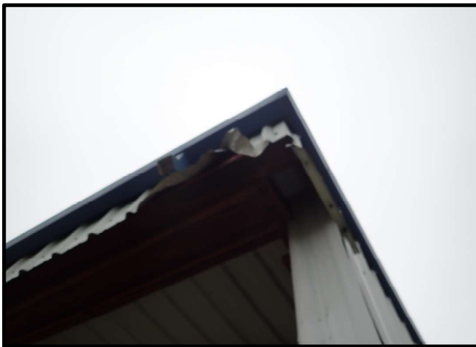
Photograph 3 - Metal wall panel damage at roof.
