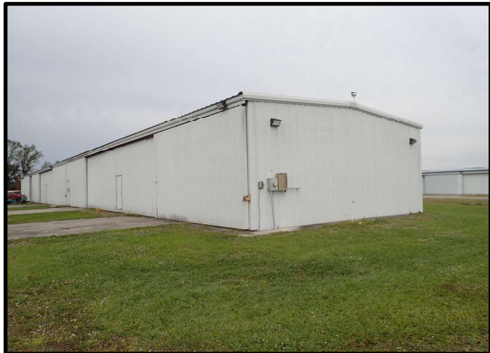
Photograph 1 - Overall view of hangar.
