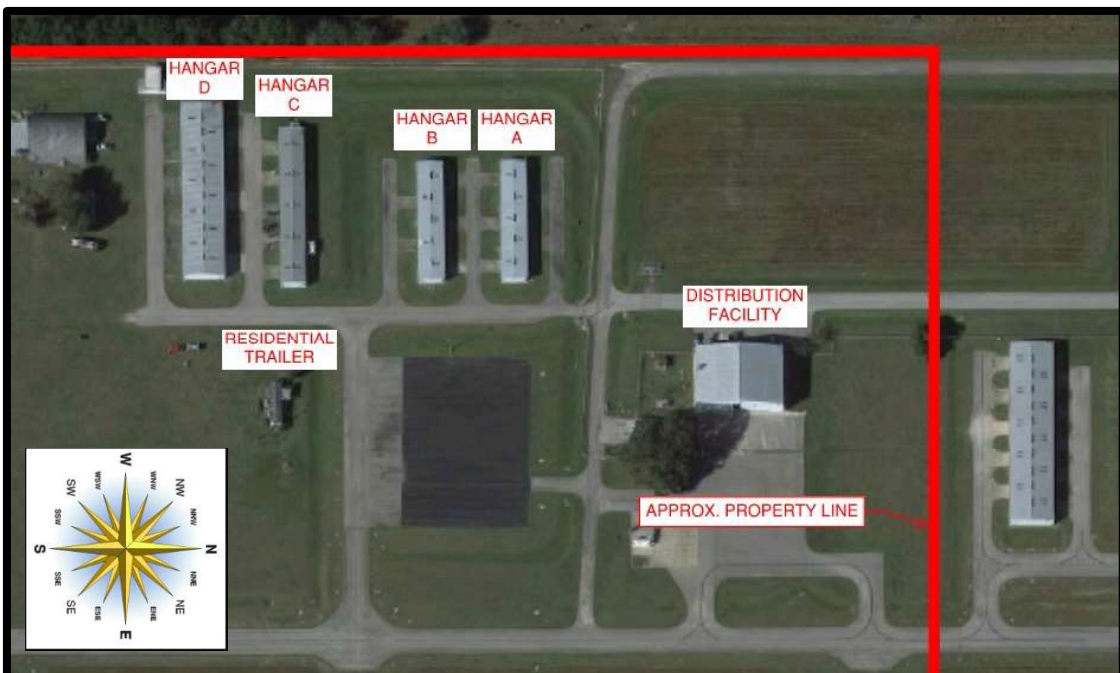
Figure 2 – (Google Earth) Aerial view of the subject property with building designations.
