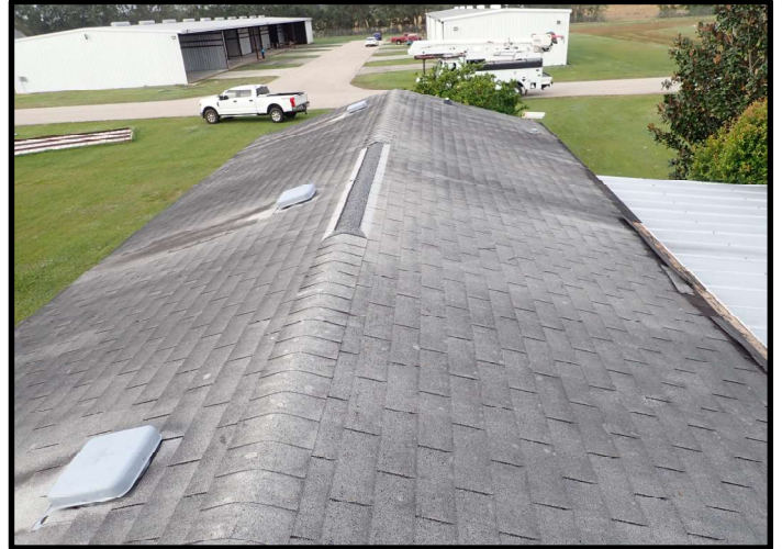
Photograph 2 - Overall view of roof.
