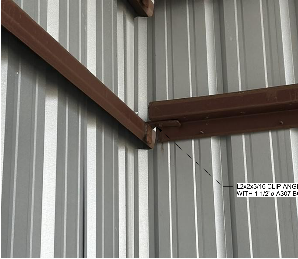
3 S905 TYP GIRT TO GIRT CONNECTION SCALE: 3/4" = 1'-0"
