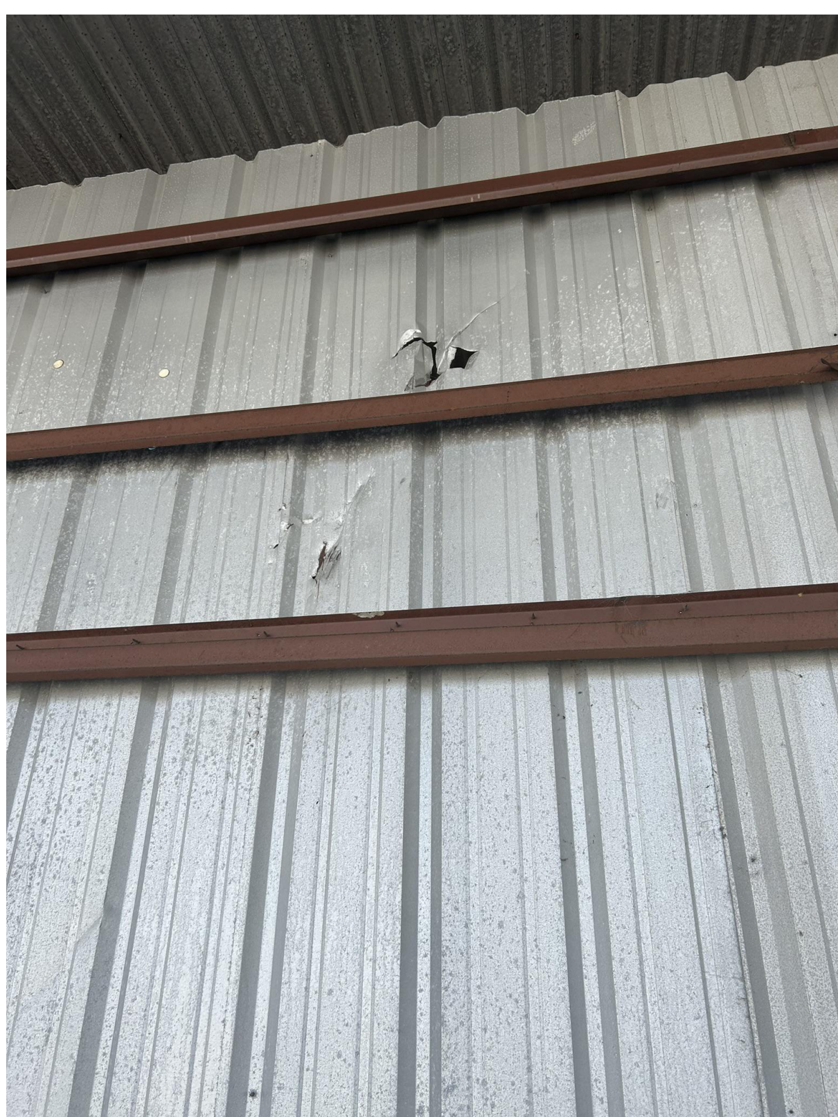
8 S900 HANGAR D DAMAGED WALL PANELS TO BE REPLACED (MULTIPLE LOCATIONS) SCALE: 3/4" = 1'-0"
