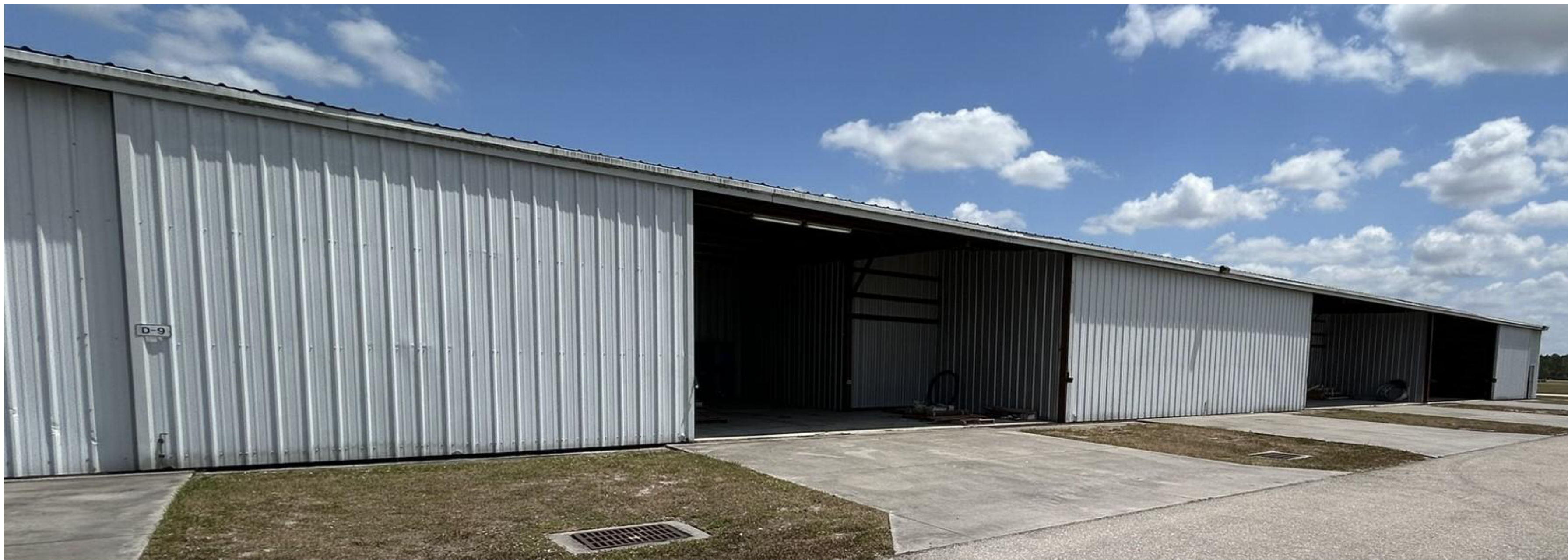
2 S900 HANGAR D REAR VIEW (5 DOORS EACH SIDE REQUIRES REPLACEMENT) SCALE: 3/4" = 1'-0"
