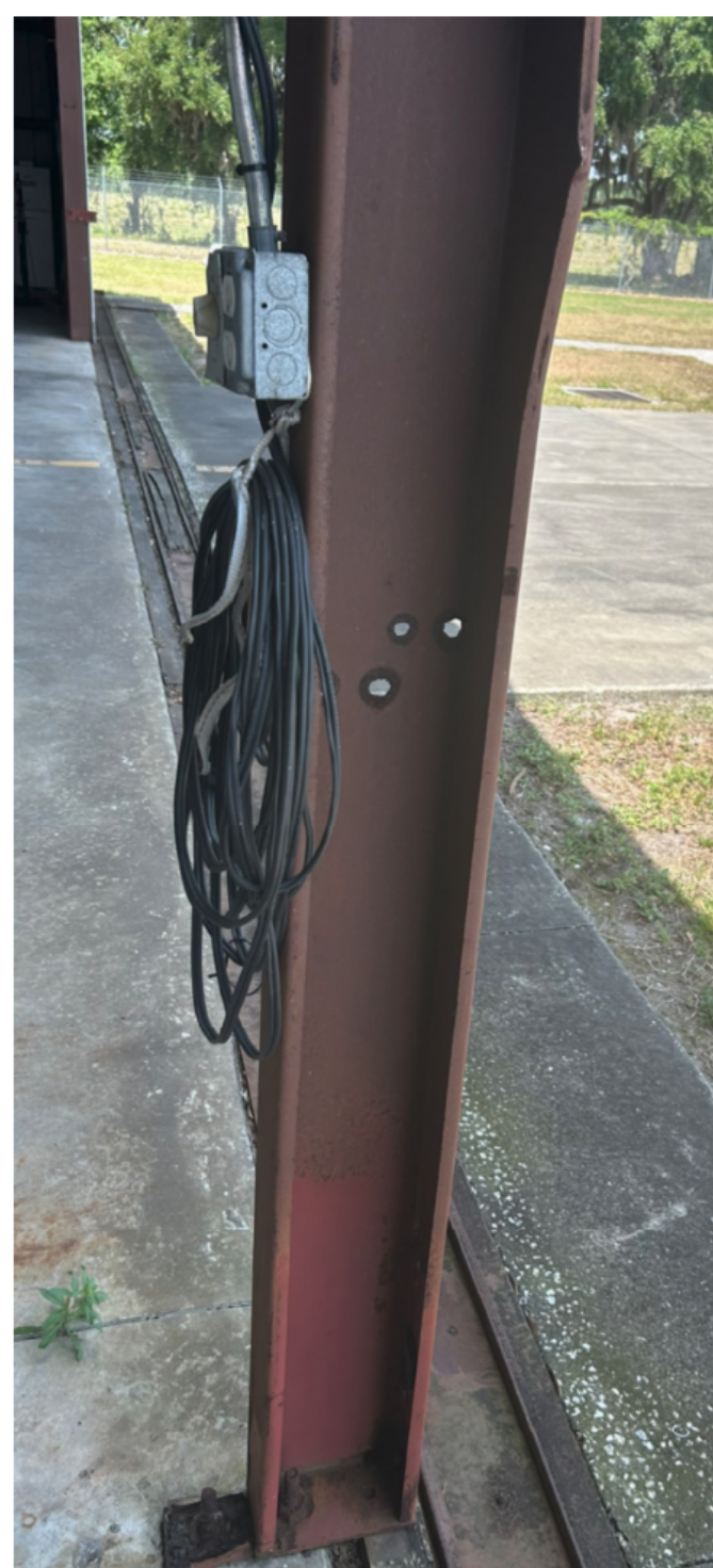
9 S900 HANGAR D DAMAGED JAMB TO BE REPLACED SCALE: 3/4" = 1'-0"
