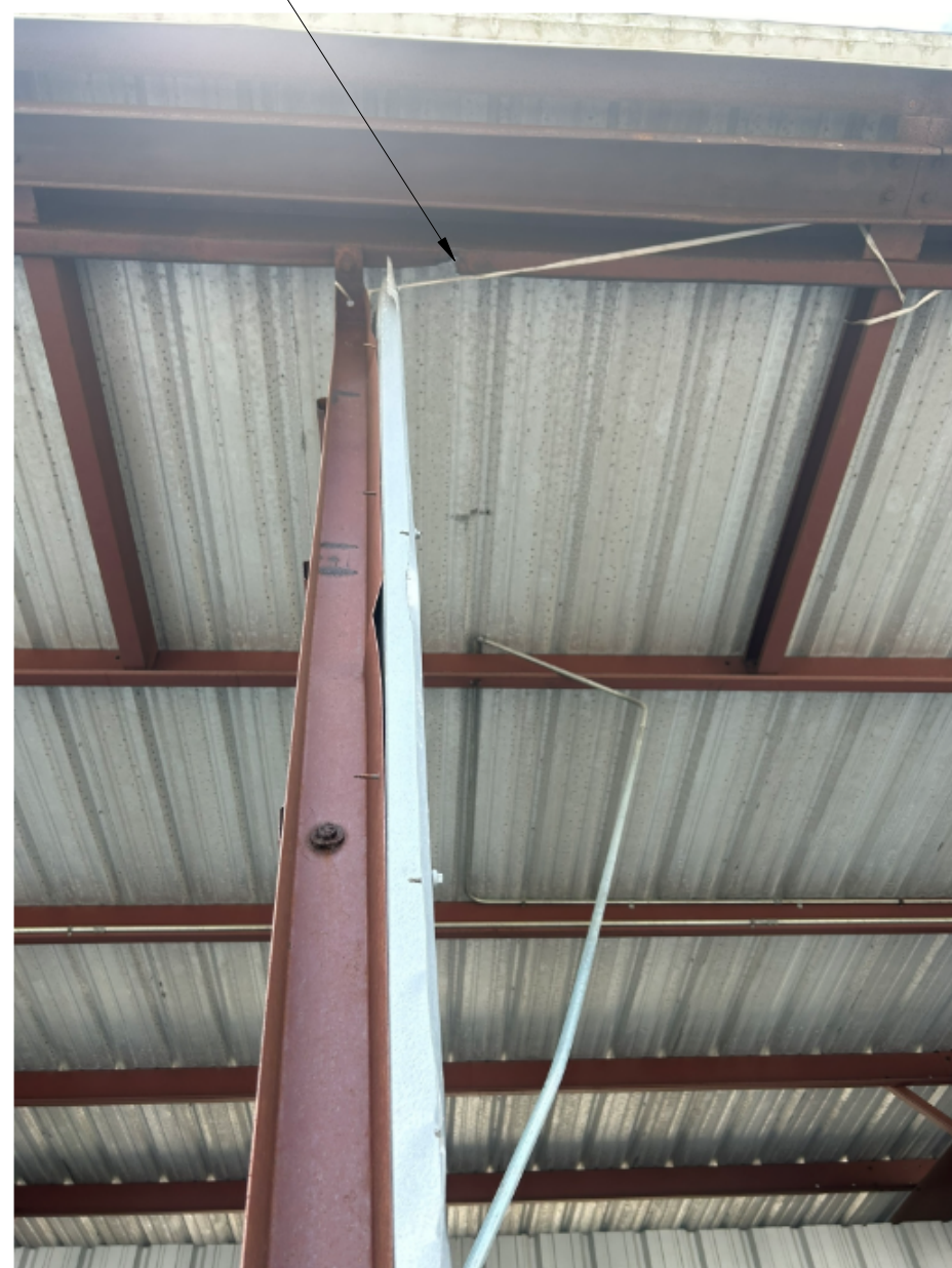
HANGAR D DAMAGED JAMB CONNECTION AT TOP (REPLACE JAMB AND DIVIDER WALL SCALE: 3/4" = 1'-0"
