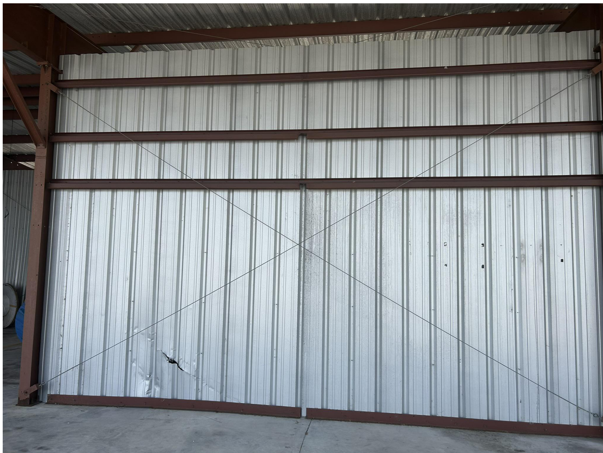
5 S900 HANGAR D DAMAGED GIRTS TO BE REPLACED (MULTIPLE LOCATIONS) SCALE: 3/4" = 1'-0"
