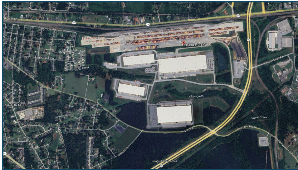
Figure 4-3: Aerial Image of Inland Port Greer
