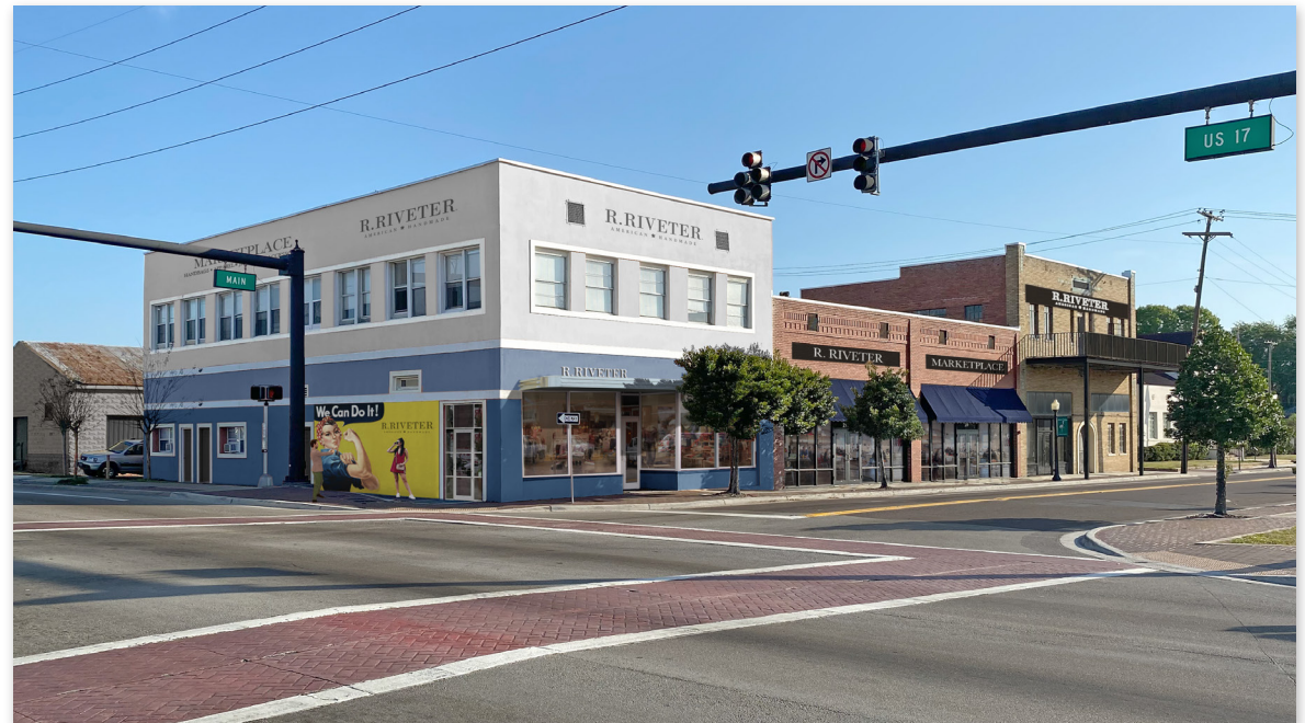
Proposed Conditions: The redevelopment of the R. Riveter complex as a business incubator could once again anchor this intersection for entrepreneurial endeavors.
