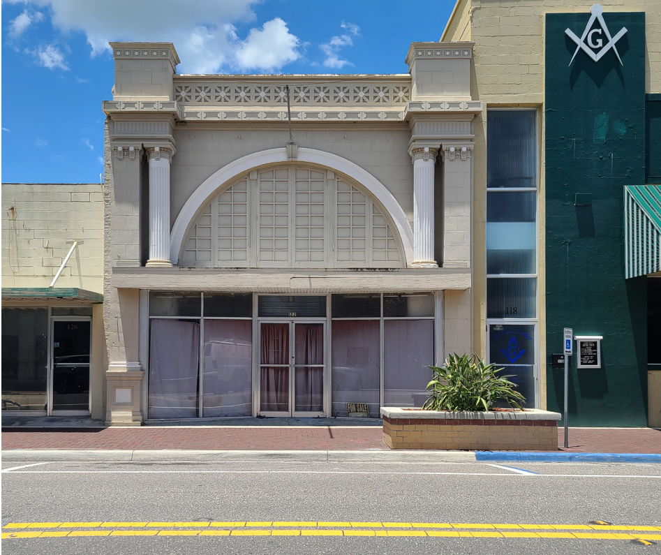
Existing Conditions: 122 West Main Street, former bank building
