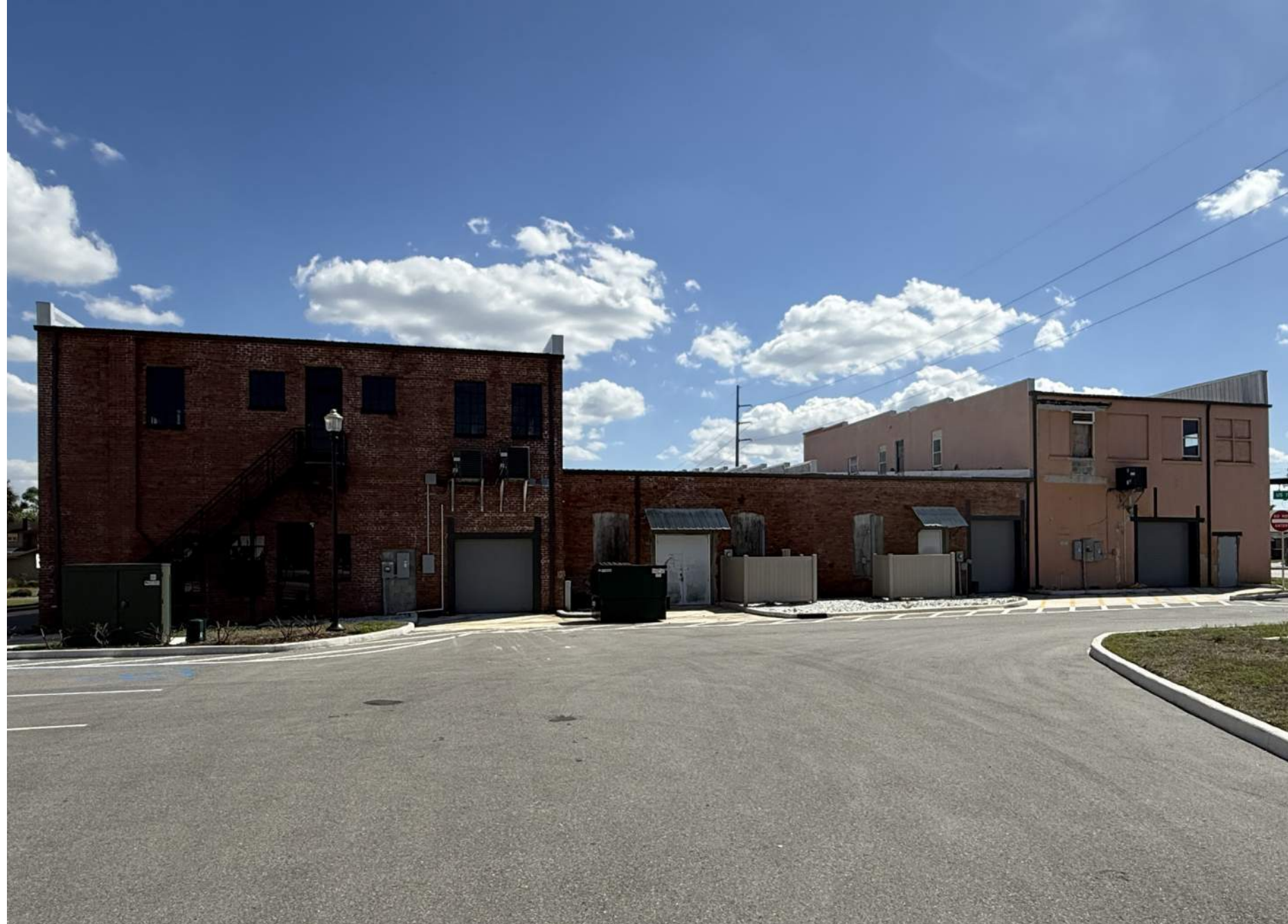
EXISTING EXTERIOR - NORTH BUILDING FACADE
