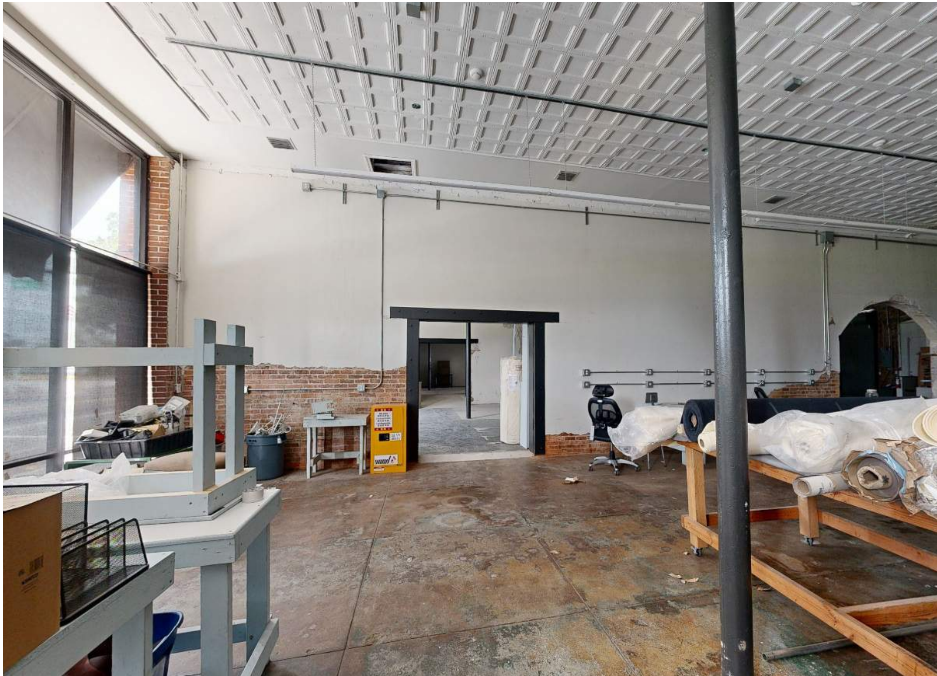
EXISTING INTERIOR - BAY 2
