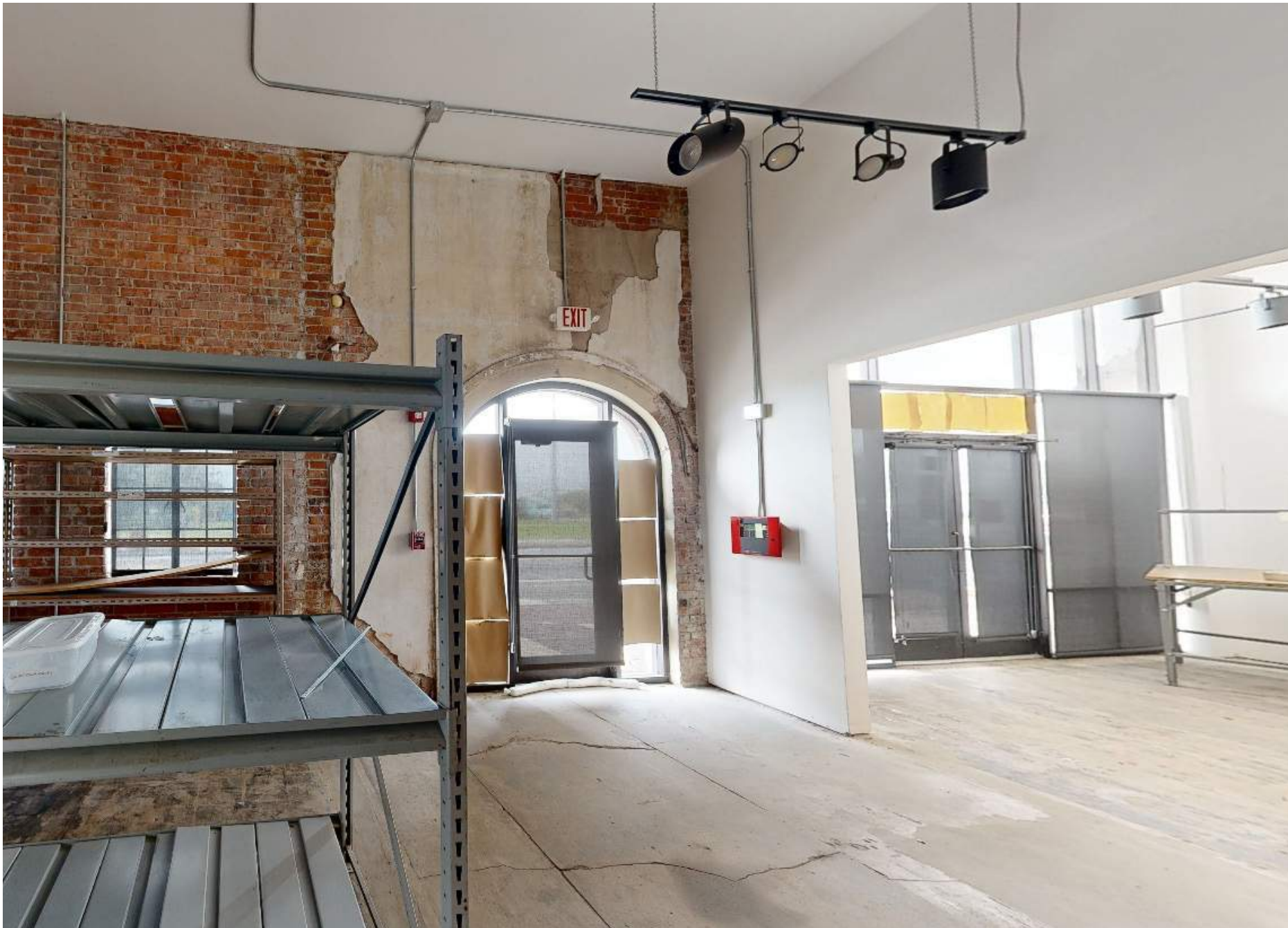
EXISTING INTERIOR - BAY 1 - LEVEL 1
