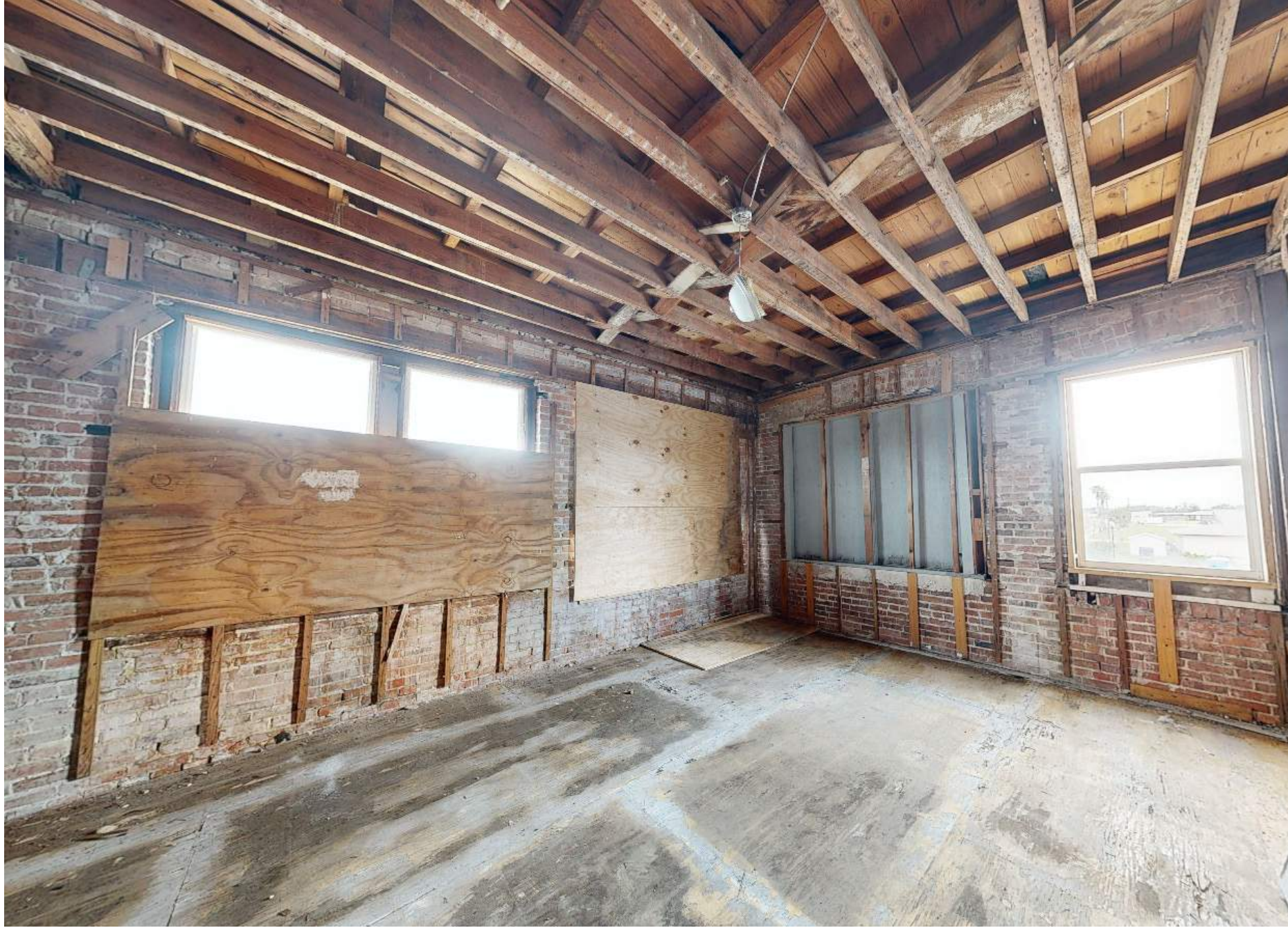
EXISTING INTERIOR - BAY 4 - LEVEL 2
