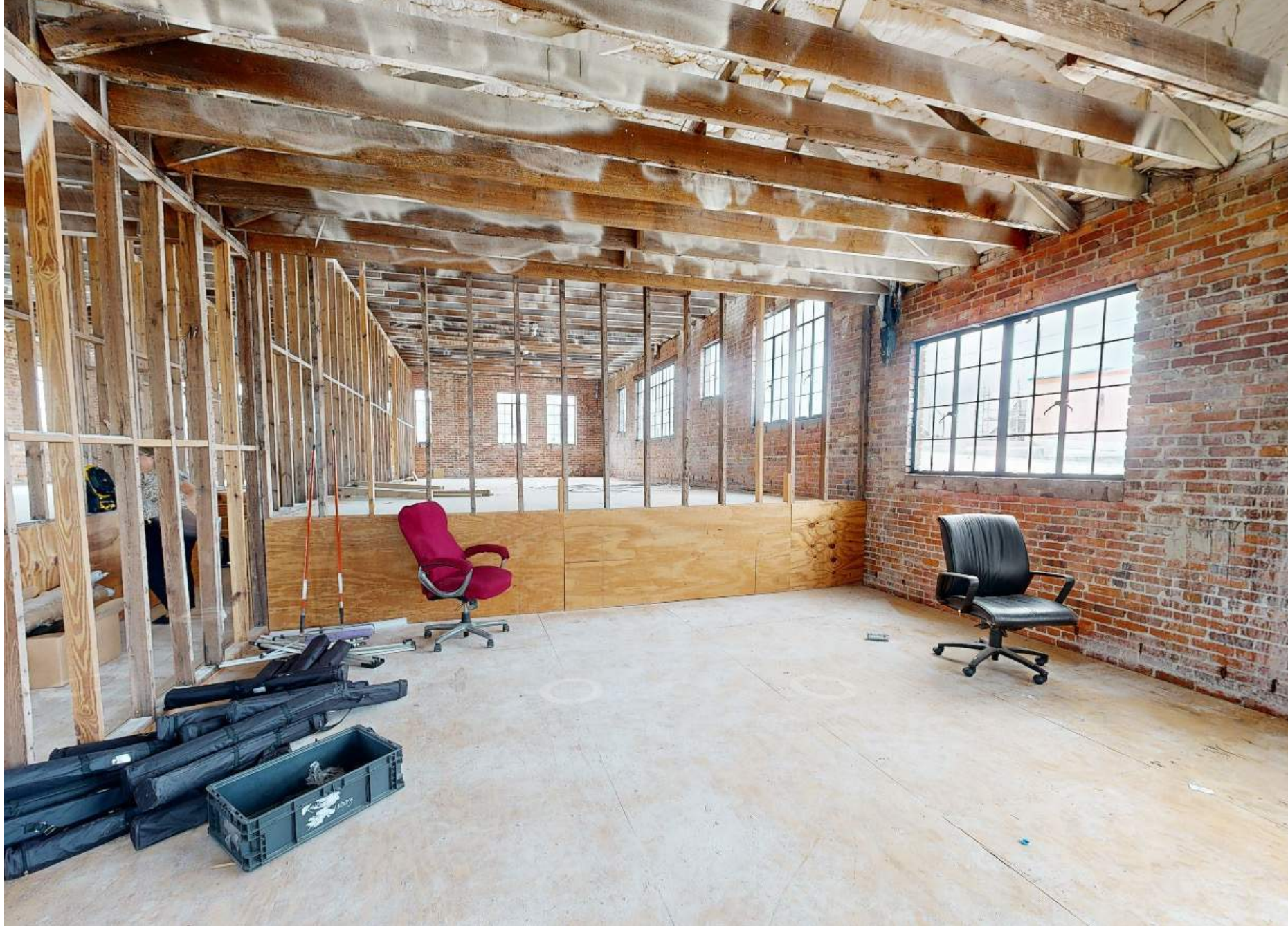
EXISTING INTERIOR - BAY 1 - LEVEL 2
