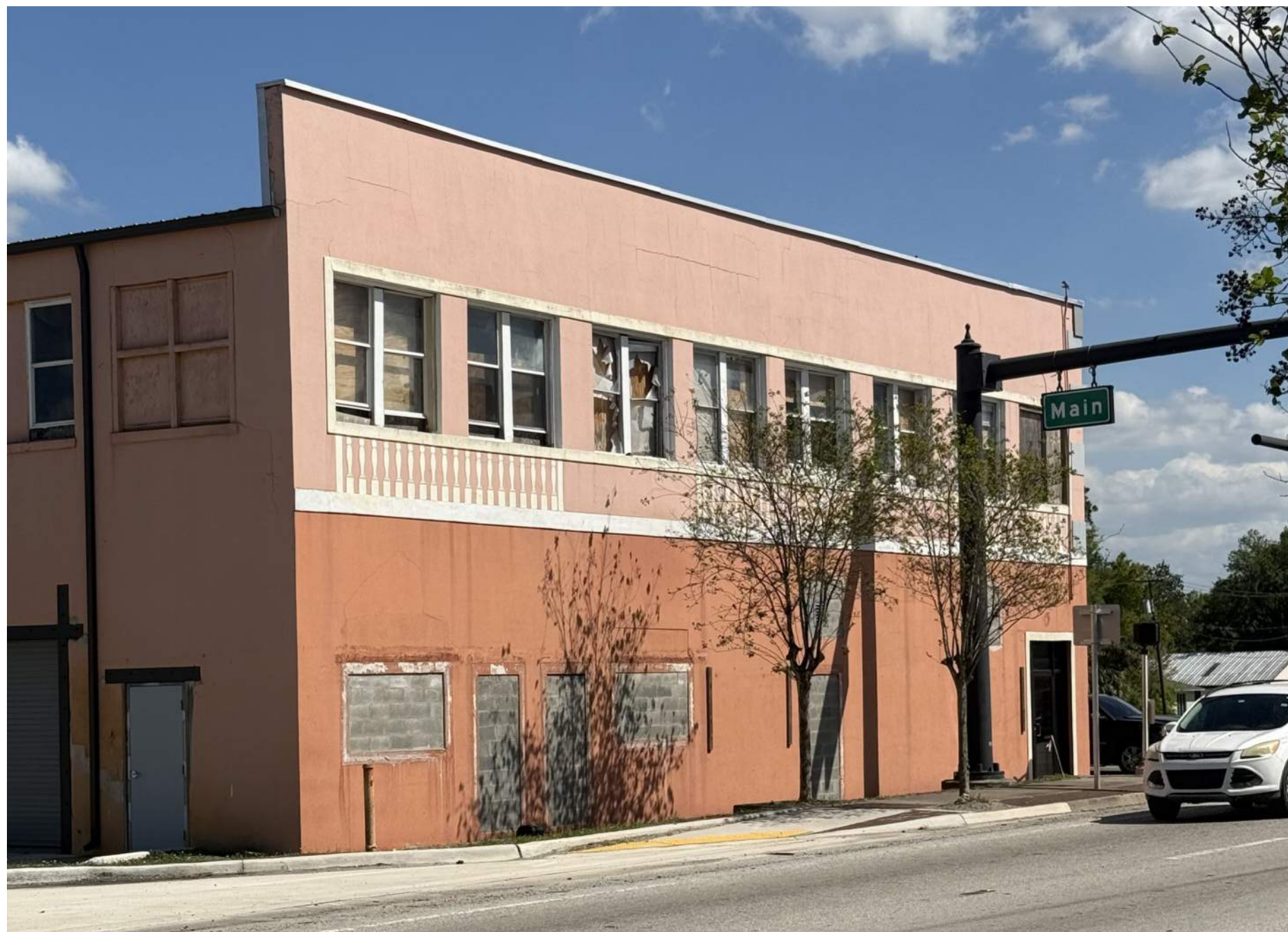
EXISTING EXTERIOR - US 17 N (BAY 4)
