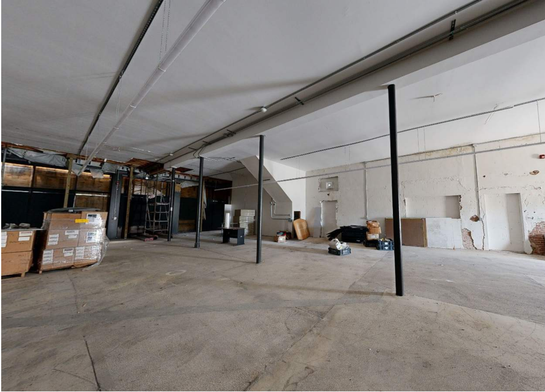
EXISTING INTERIOR - BAY 4 - LEVEL 1
