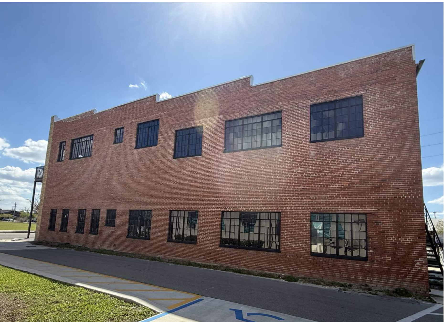
EXISTING EXTERIOR - EAST BUILDING FACADE (BAY 1)
