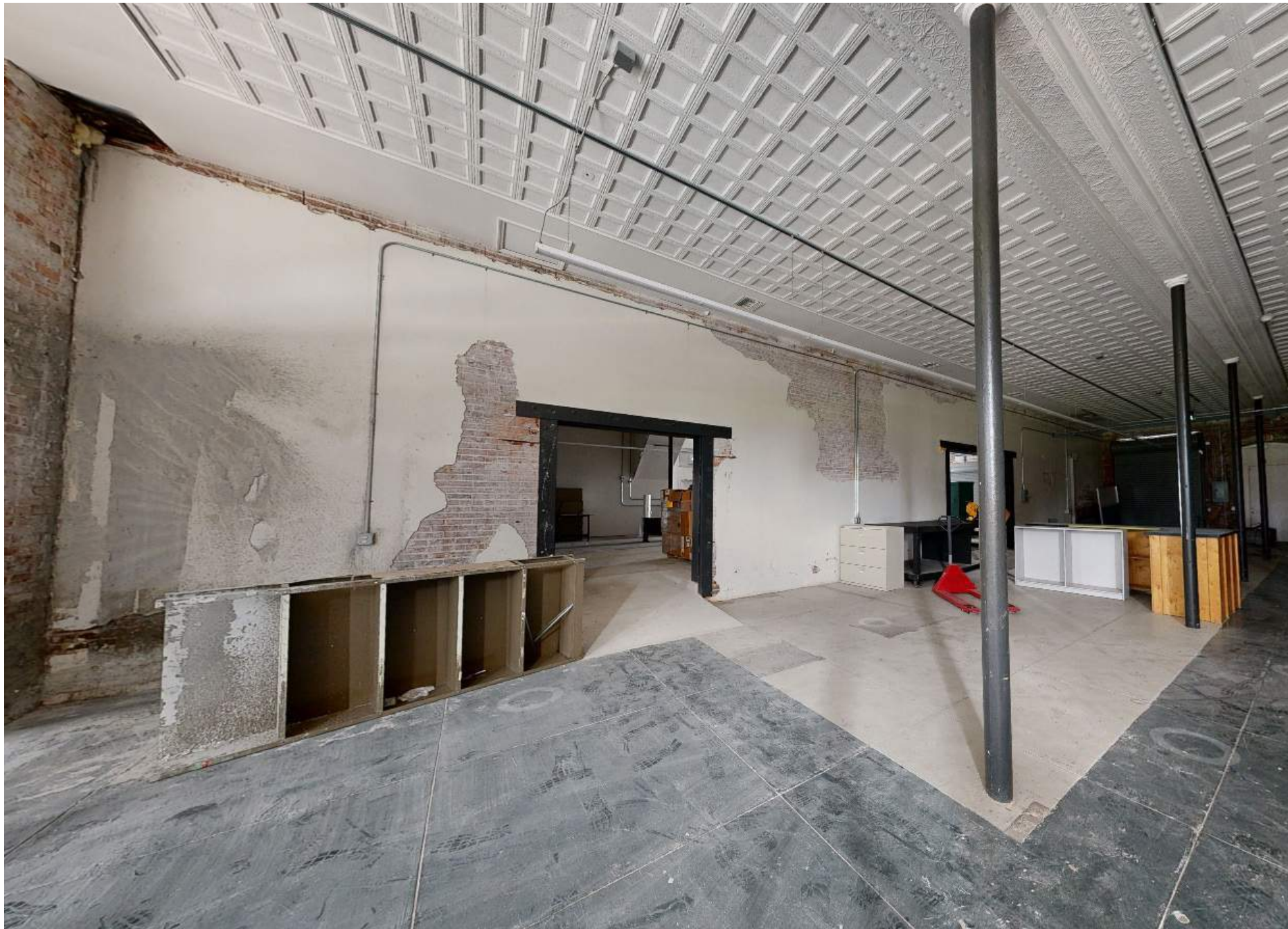
EXISTING INTERIOR - BAY 3
