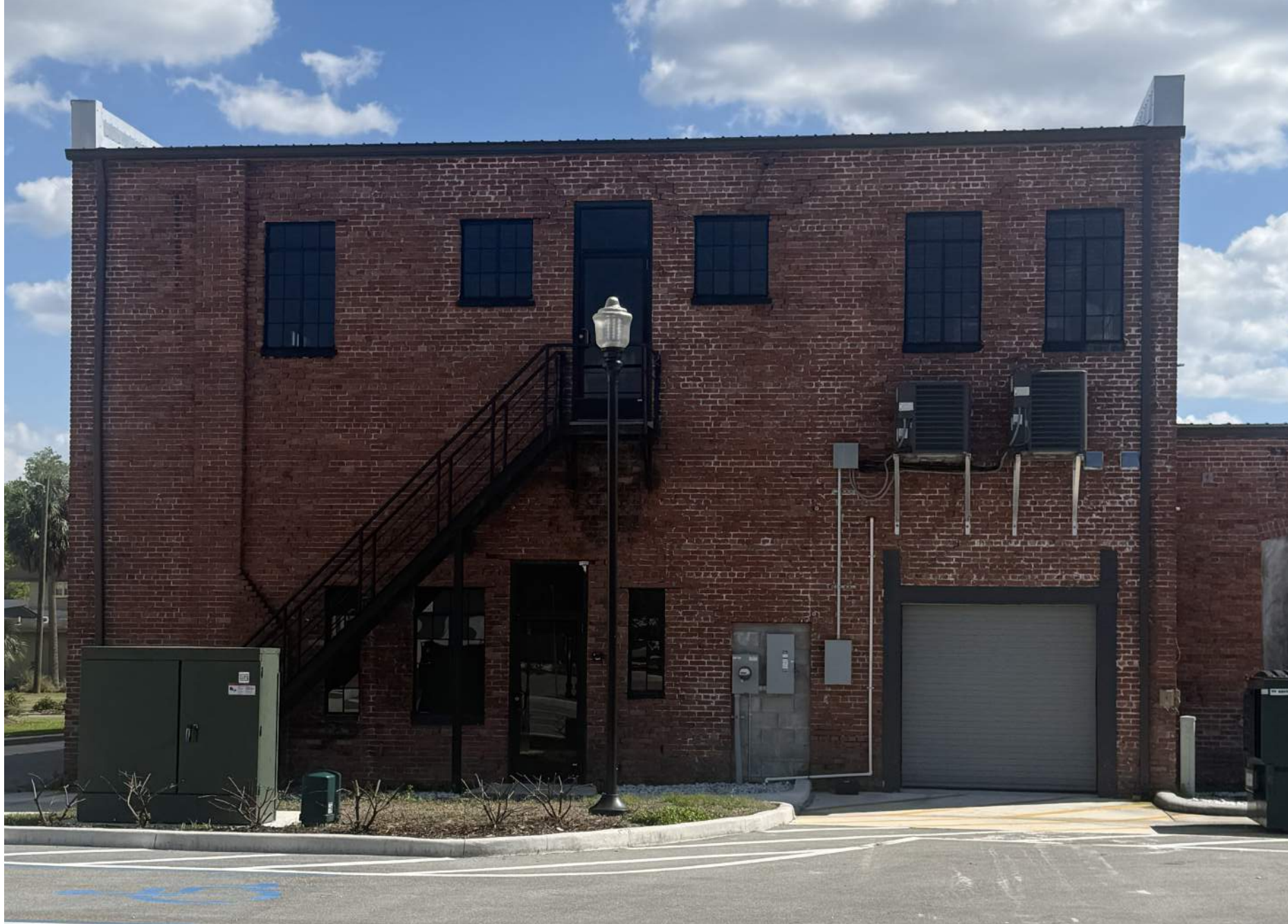
EXISTING SITE - NORTH BUILDING FACADE (BAY 1)
