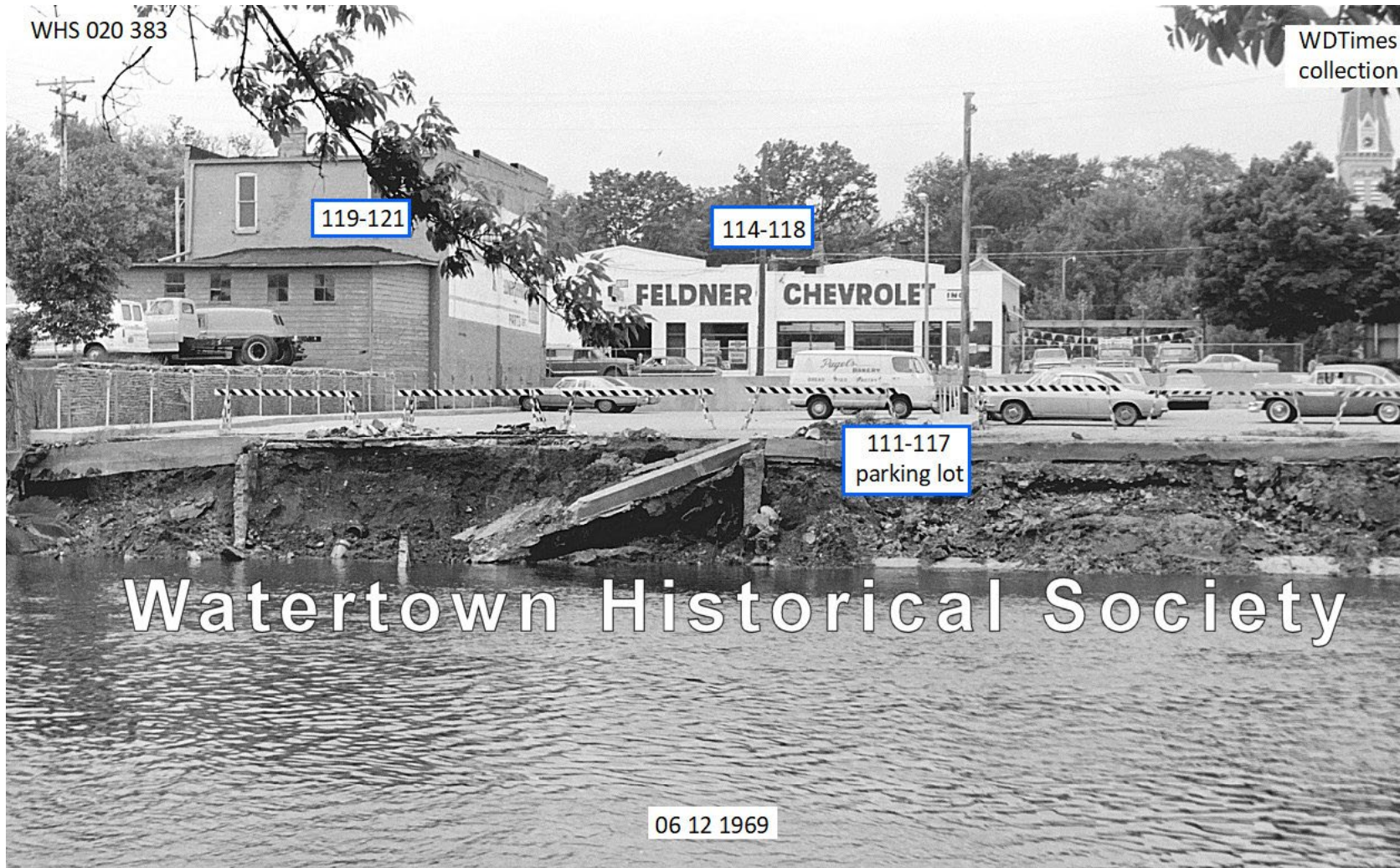
Erosion of Retaining Wall, S. Water Street Parking Lot
