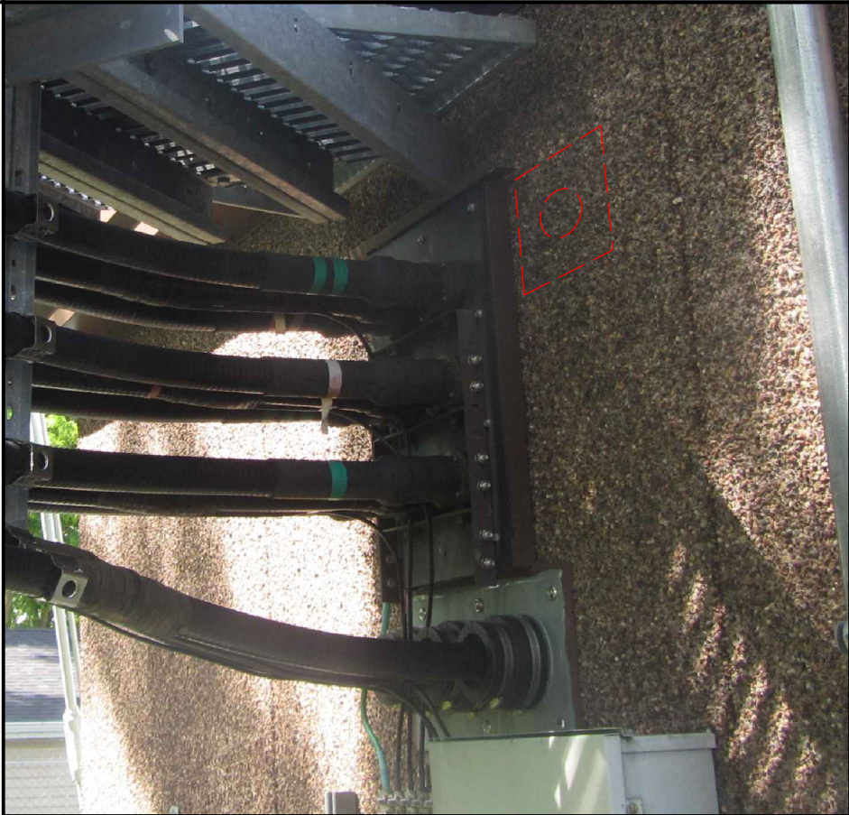
EXISTING COAX ENTRY PORT - EXTERIOR
