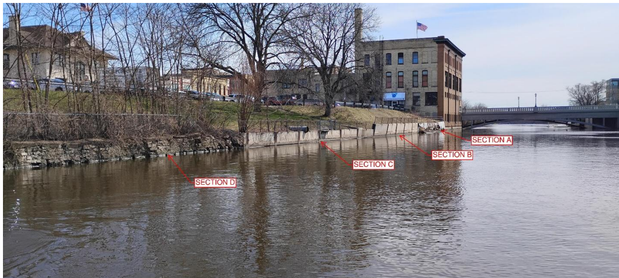
Figure 1. Each section of seawall along the east bank of the Rock River.
