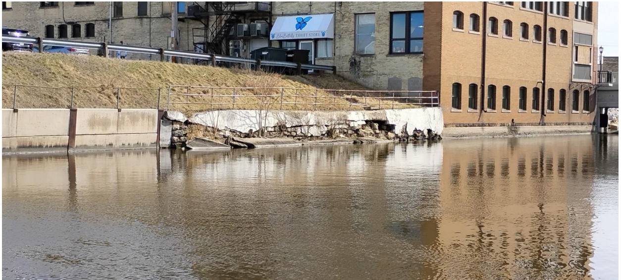
Figure 2. View of Section A looking southeast.
