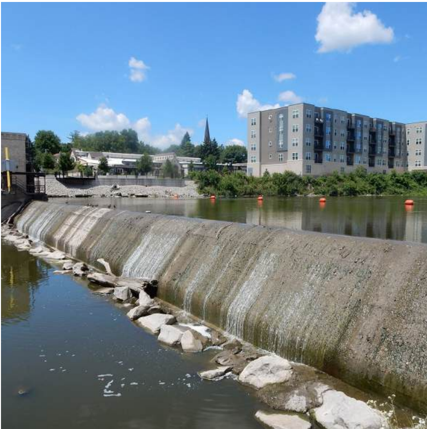
Rock River - Lower Dam
