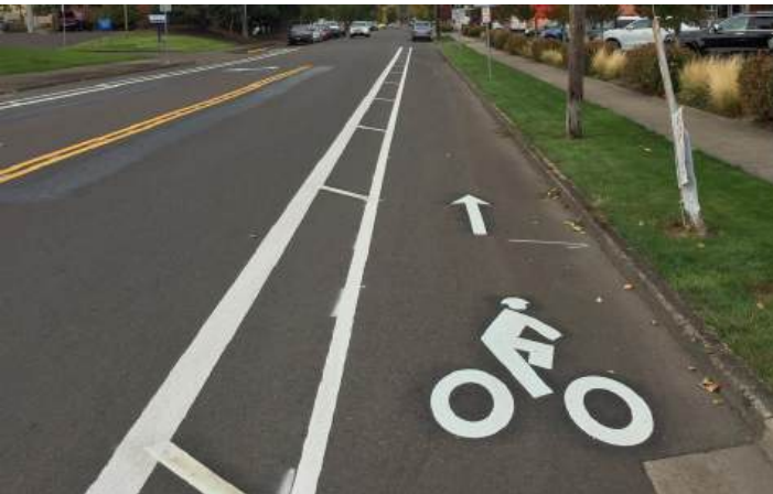
Bike Lane Example with buffered stripe markings
