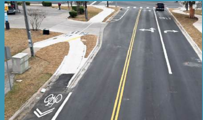
Curb ramp from on-street bike lane
