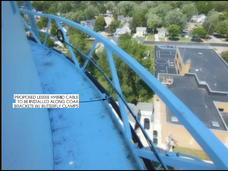
EXISTING CATWALK RAILING
