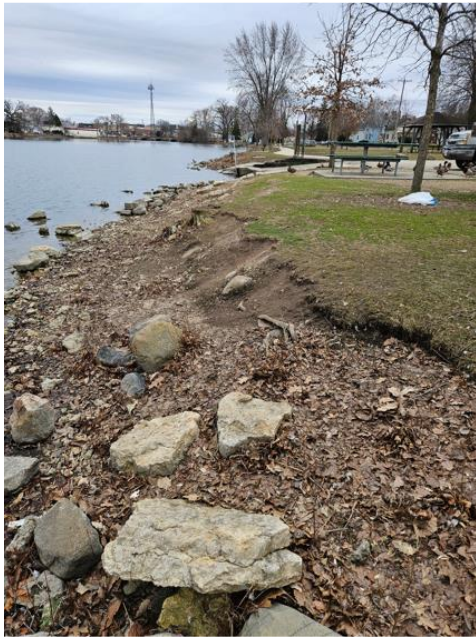
Photo 2 (facing south along shoreline) near parking lot.
