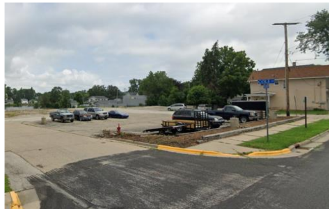
Figure 6: Current Site Conditions
