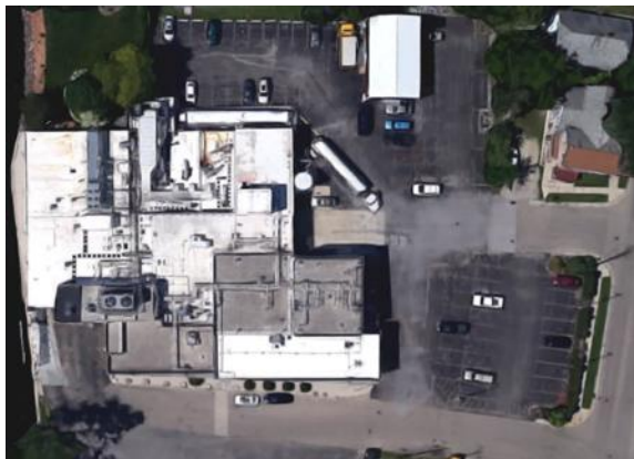
Figure 5: Aerial of Past Plant
