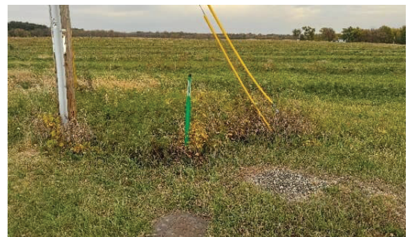
Existing MH 23A-091 at Milford/Commerce looking east towards the WWTP.
