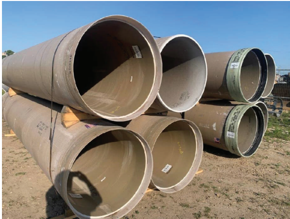
Thirty-six-inch Hobas FRP Sanitary Sewer.
