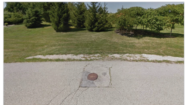
Existing MH 23B-004 looking west towards the proposed sewer alignment.
