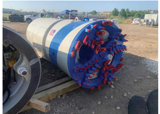
Forty-eight-inch microtunneling machine used for steel casing installation beneath CPKC railway.
