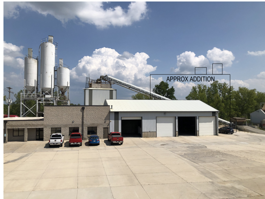
EXISTING WEST ELEVATION PHOTO
