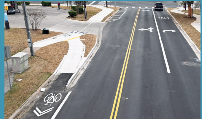
Curb ramp from on-street bike lane
