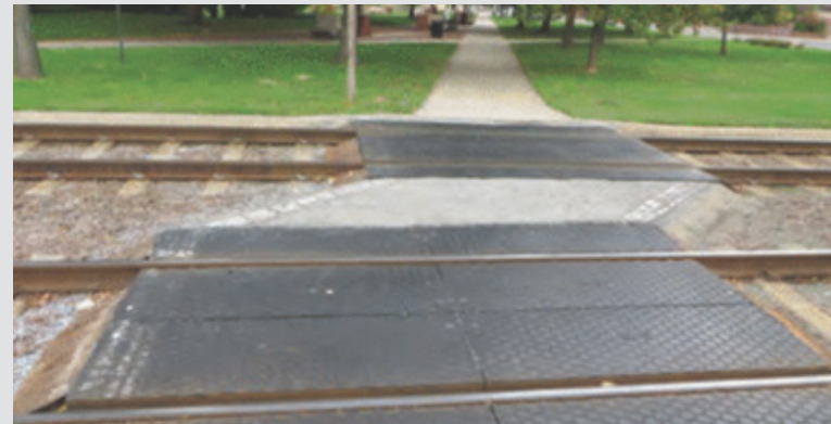
An example of a pedestrian trail-rail crossing with sufficient surface materials, Transportation Research Board.
