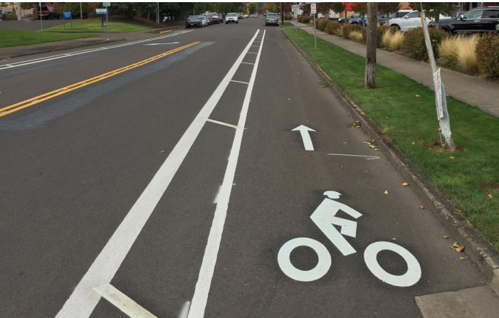
Bike Lane Example with buffered stripe markings
