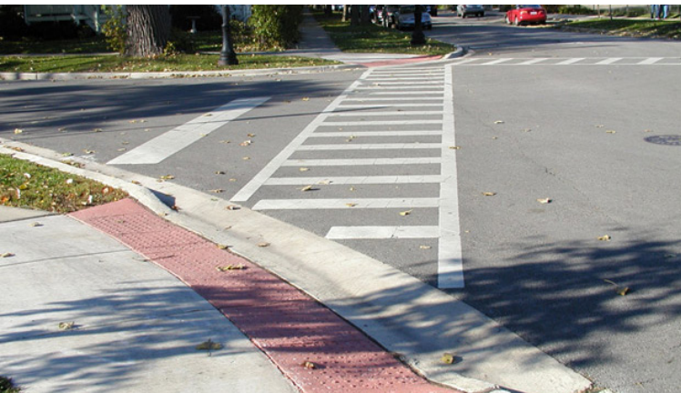
Curb ramp with crosswalk markings
