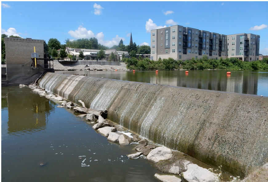
Rock River - Lower Dam
