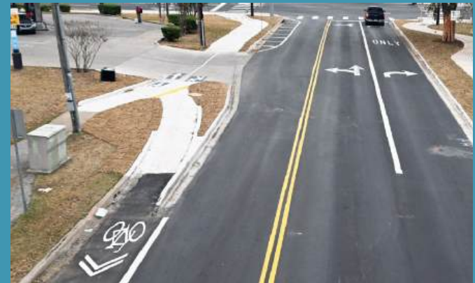
Curb ramp from on-street bike lane
