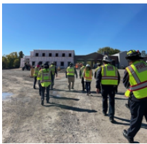
WFD Staff toured the progress of the new station
