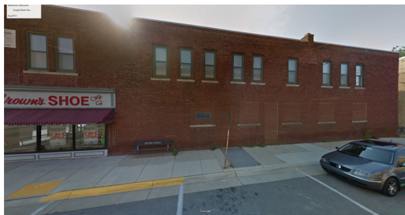
EXISTING STREET VIEW
