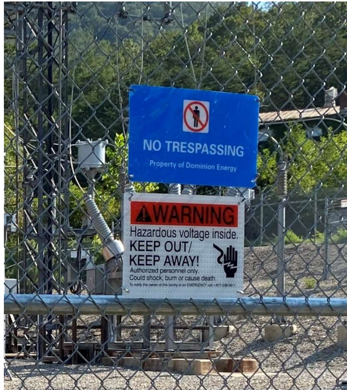
Picture 1 - Example photo of substation perimeter fence signage.
