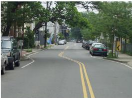
Creating a traffic calming chicane by switching parking to alternate sides.
