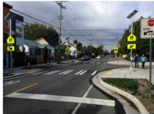
This Rectangular Rapid Flashing Beacon installation is at a school crossing on a busy neighborhood street in Seattle.
