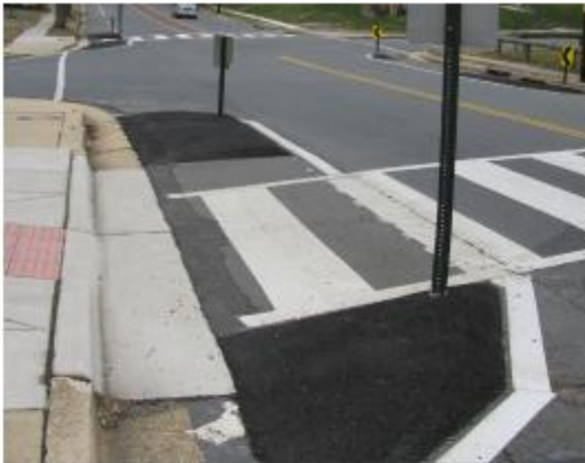
Temporary bulb-outs at an intersection in Alexandria, VA
