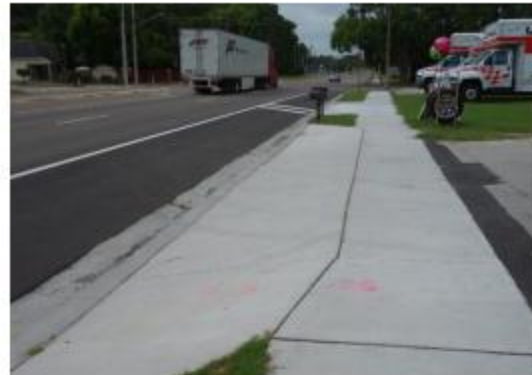
This section of new sidewalk on a major road in Jacksonville, FL maintains a level surface for the sidewalk and a more steeply sloping driveway apron for motor vehicle access.
