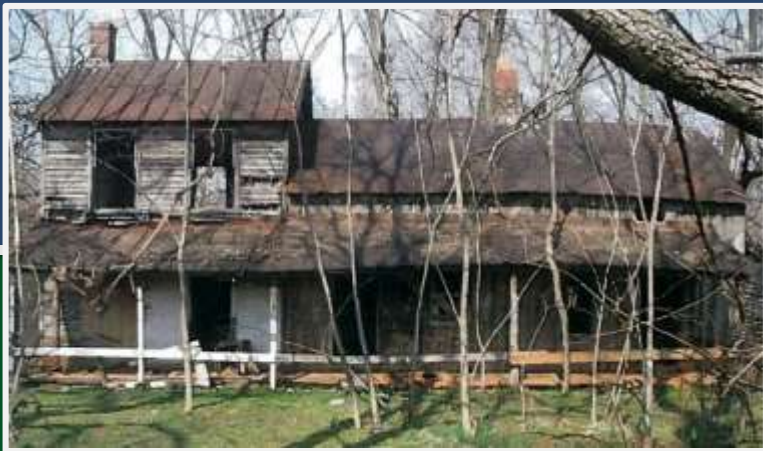
Leeton Forest log house w/two-story additions (ca. 1830 log portion, ca. 1870 & 1920 two-story additions)
