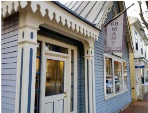
Figure 3-4: This building uses two colors of paint to draw attention to the building's quaint and intricate detailing.
